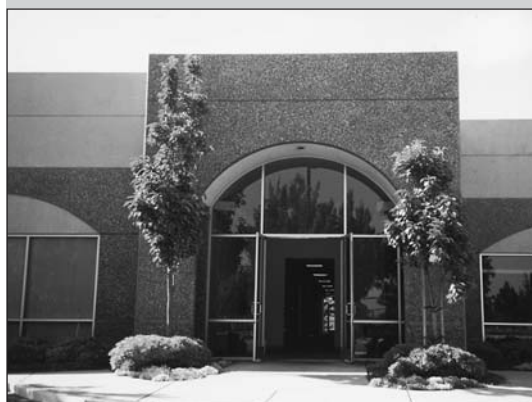
The Division of Intercollegiate Athletics is housed in the Alan B. Simpkins Intercollegiate Athletics Administration Building. The street address is 1393 S. 7th Street, next to the corner of 7th and Alma.
