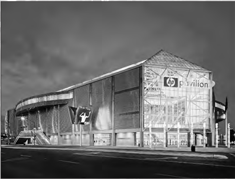
HP Pavilion - Home of the San Jose Sharks
