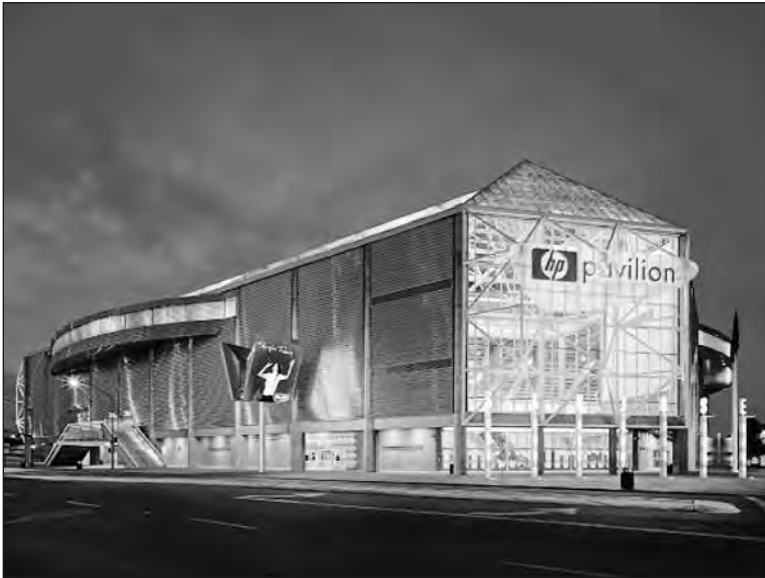
HP Pavilion - Home of the San Jose Sharks
