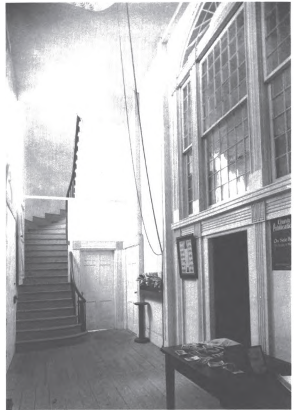
2-14. Vestibule, Kirtland Temple, looking south. The door built into the the stair kept small children from going upstairs while worship services were being held in the lower court. (In this view, the door is open and against the wall on the left.) Photographed by Carl F. Waite, April 1934.
