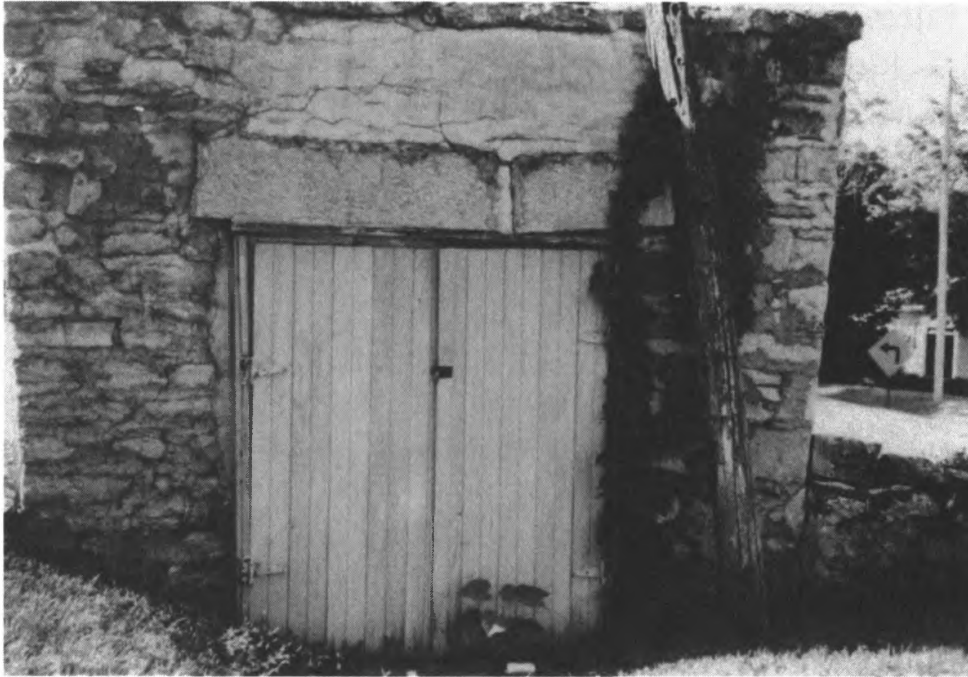
Figure 6. Wine cellar on Warsaw Street.
