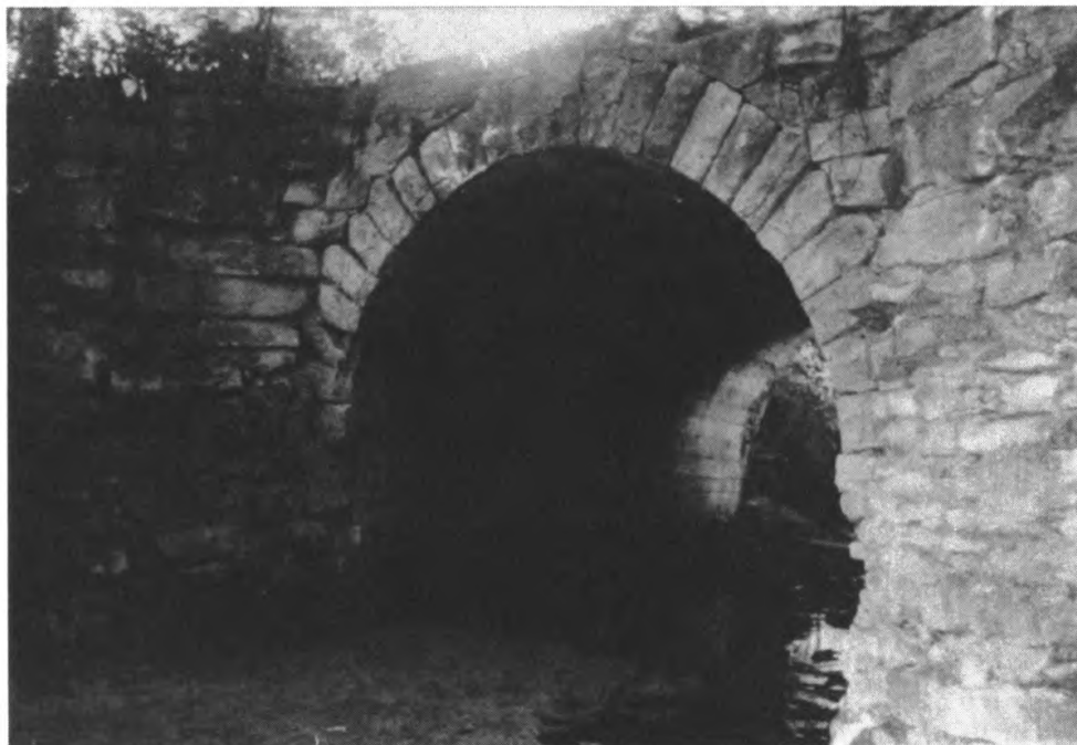
Figure 5. Stone arch bridge.
