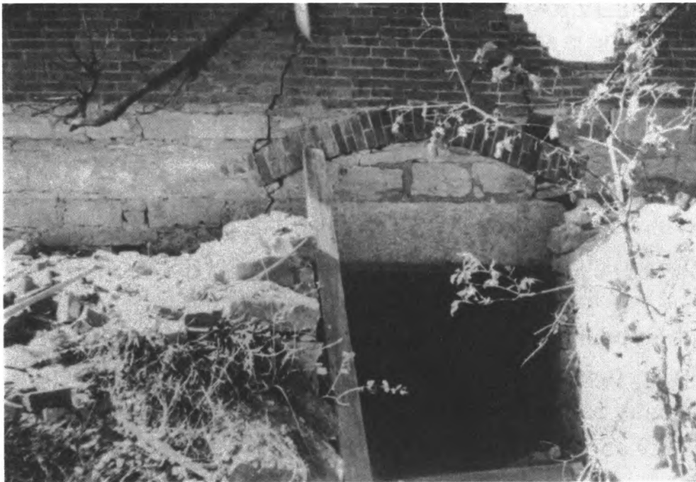
Figure 8. Wine cellar on Winchester Street.
