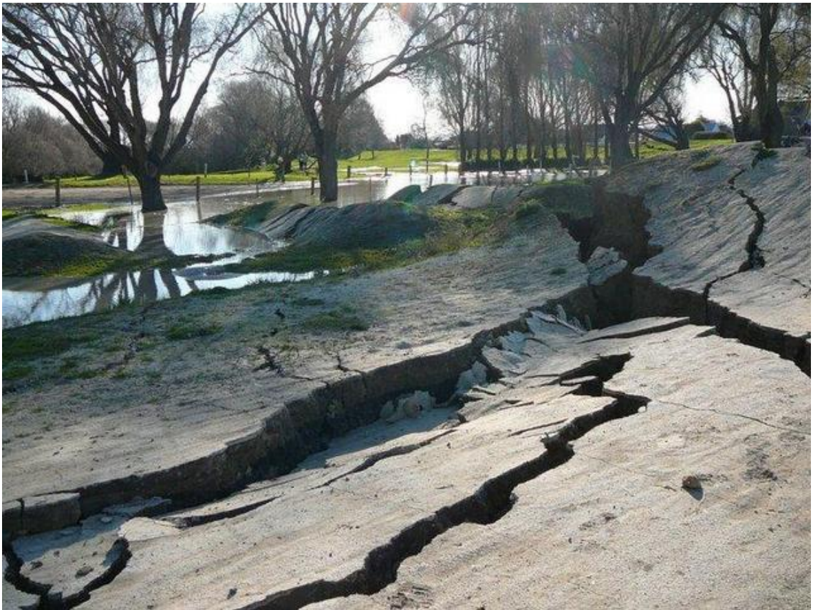
Figure 52. Lateral spreading caused by October 2013, 7.1 magnitude earthquake in Bonol, Philippines (courtesy AFP News, 2013; LDE, Ltd., 2014)
