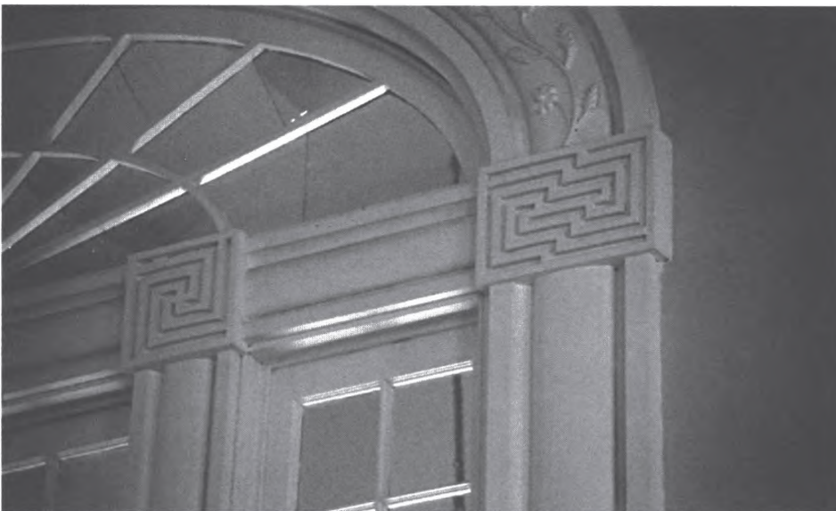
5-21. Two Greek frets on the east window, upper court. Note how the more common fret on the left has been modified on the right by extending it to a rectangular format, creating a new diagonal axis through the design. Compare the moldings to fig. 5-11.
