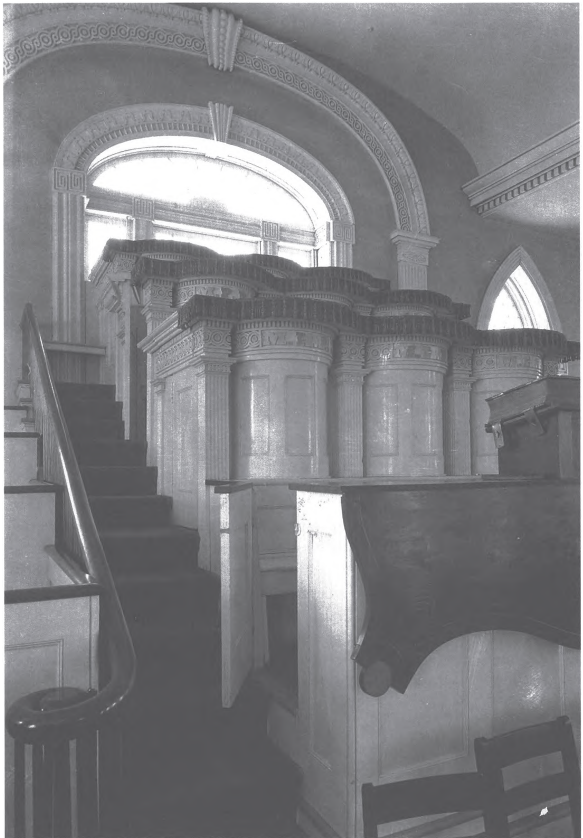
5-3. Pulpits and west window, lower court. Fringed covers on the pulpits covered the graffiti-scarred tops until their sanding and refinishing in the 1960s. The upper arch is composed of egg-and-dart, bead-and-lozenge, and running-guilloche moldings. The lower arch has opposed Vitruvian scrolls and a series of transversely oriented half-round moldings. Photographed by Carl F. Waite, April 1934.
