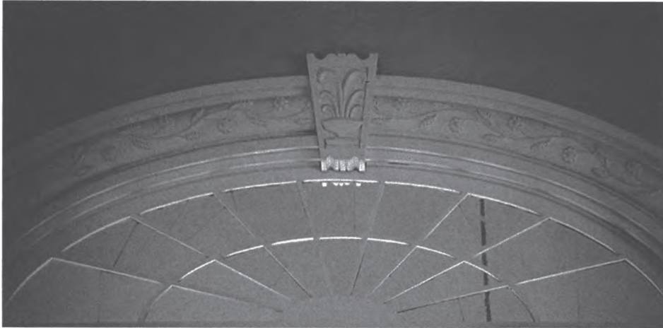
5-19. An arch with an intricate, carved, running-vine motif. East window, upper court. Designed by Truman Angell.
