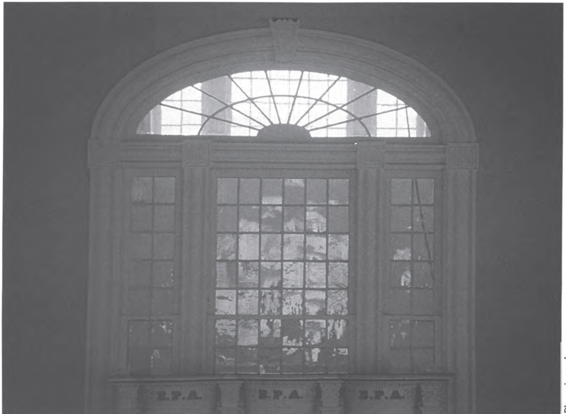
5-9. East window, lower court. Light from the exterior window, visible through the fanlight, was a source of illumination for the lower court.
