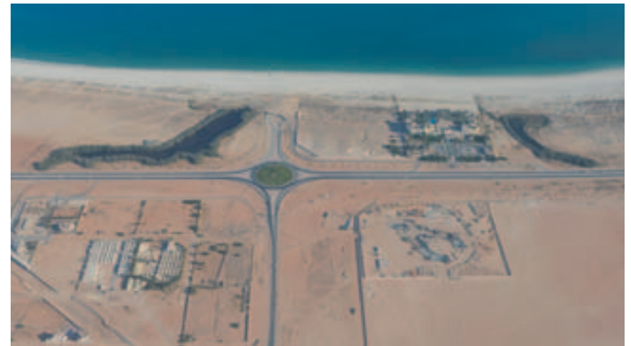
This aerial view shows Qurms As Saghir and Al Kabir with the Hilton hotel between them.
