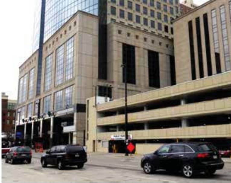
Figure 9: Third Street at Berning Place, Cincinnati, Ohio, March 2014.
