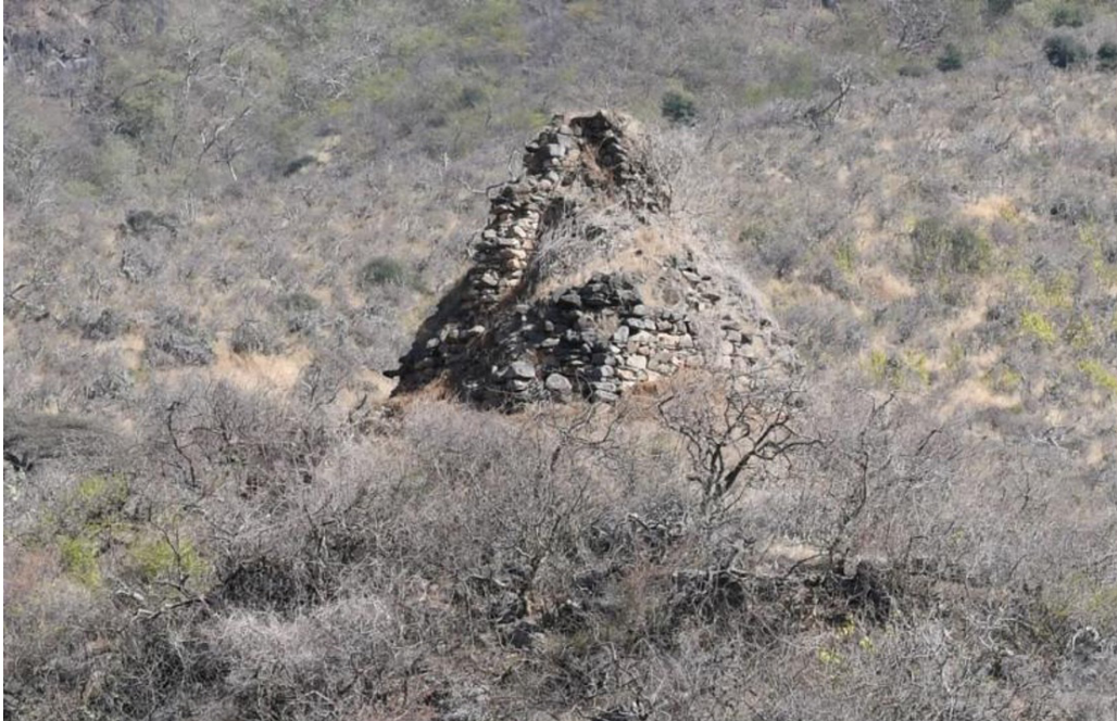
Figure 3. The tower on the al Hauta coast. It stands 6 meters (just over 20 feet) tall.
