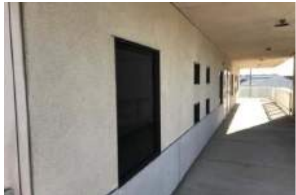
#12 EXTERIOR WALL, PAINTED SURFACE
