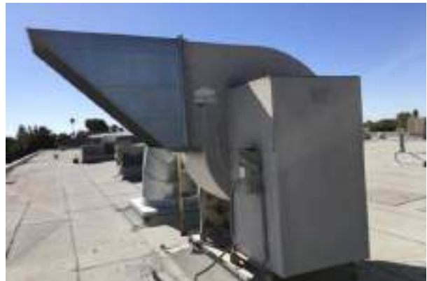
#48 EXHAUST FAN, CENTRIFUGAL
