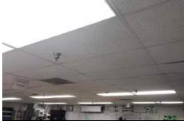
#20 INTERIOR CEILING FINISH, SUSPENDED ACOUSTICAL CEILING TILE (ACT)
