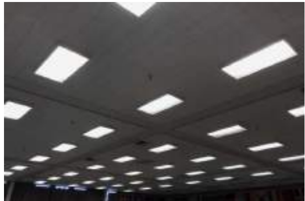
#18 INTERIOR CEILING FINISH, HARD CEILING TILE
