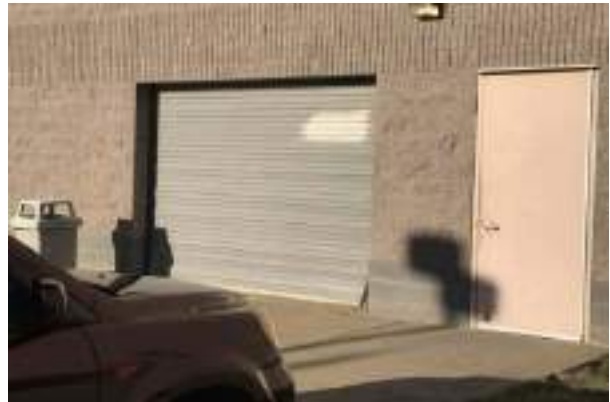
#10 EXTERIOR DOOR, OVERHEAD DOCK DOCK
