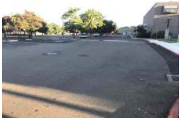
#82 PARKING LOTS, ASPHALT PAVEMENT, SEAL & STRIPE
