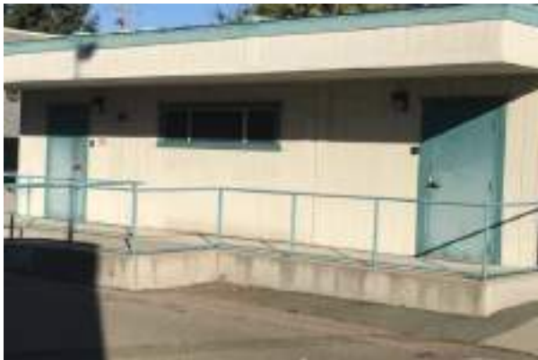
#11 EXTERIOR DOOR, STEEL
