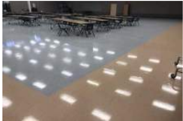
#22 INTERIOR FLOOR FINISH, VINYL COMPOSITE TILE (VCT)
