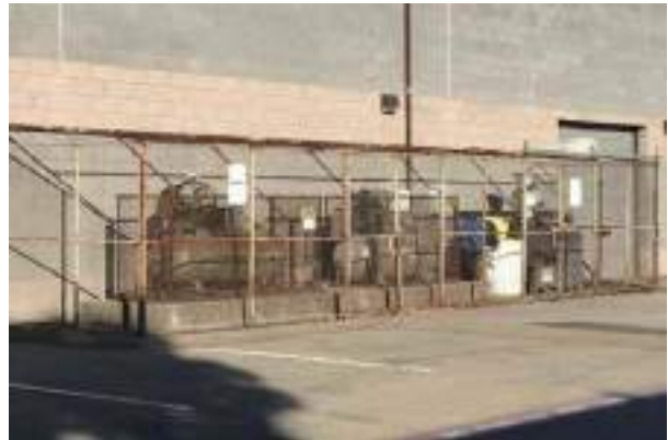
#4 DEFICIENCY FENCES & GATES, CHAIN LINK
