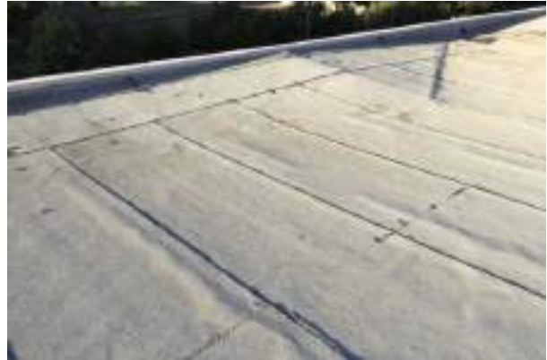
#14 ROOF, BUILT-UP MEMBRANE
