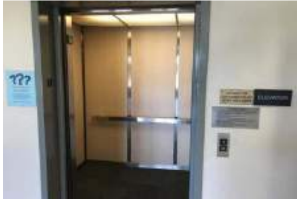
#31 ELEVATOR, INTERIOR FINISHES
