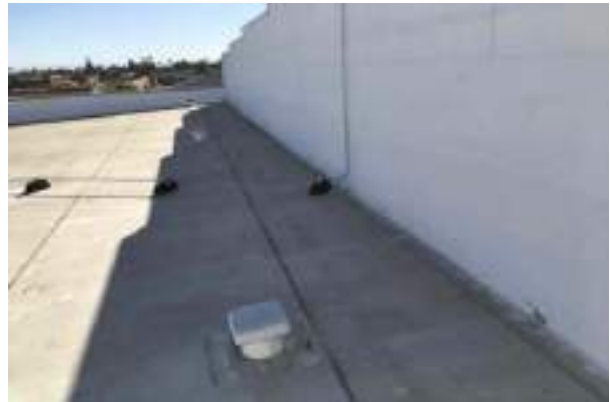
#16 ROOF, TPO/PVC MEMBRANE
