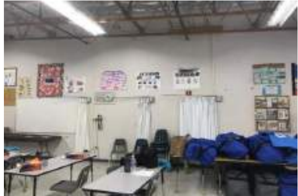
#26 INTERIOR WALL FINISH, PAINTED SURFACE
