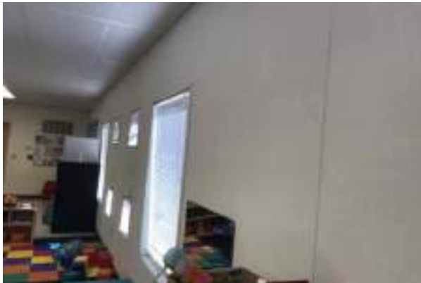
#27 INTERIOR WALL FINISH, VINYL PANELING
