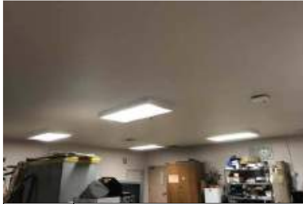
#19 INTERIOR CEILING FINISH, PAINTED SURFACE
