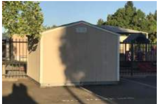
#90 SHED, WOODEN FRAMED
