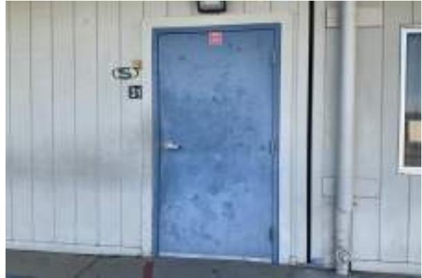
#14 EXTERIOR DOOR, STEEL
