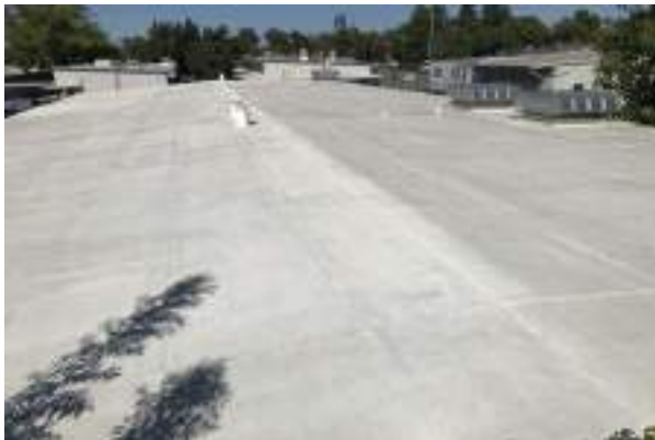
#11 MODIFIED BITUMINOUS ROOFING
