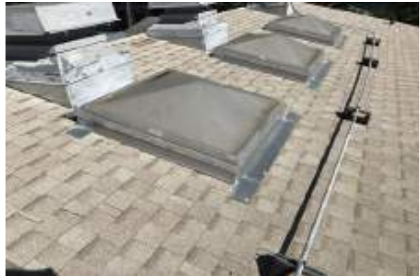
#10 ASPHALT SHINGLES AND SKYLIGHT
