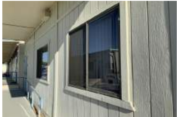
#16 WOOD SIDING AND ALUMINIUM WINDOWS
