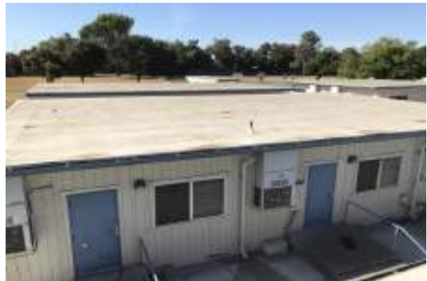
#12 PVC/TPO ROOFING
