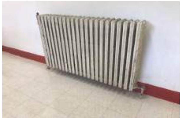
#54 BUILDING A RADIATOR, HYDRONIC
