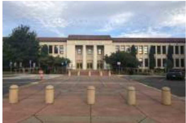
#4 FRONT ENTRANCE OF BUILDING A
