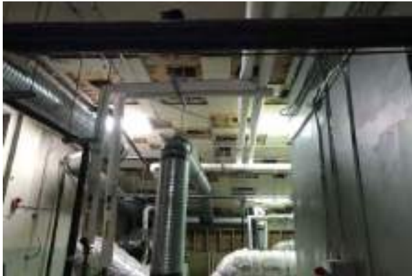
#47 BUILDING C ATTIC SPACE
