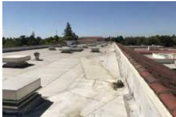
#18 ROOF OF BUILDING A
