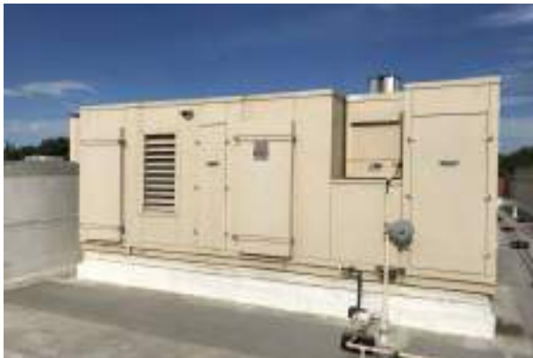
#53 BUILDING A PACKAGED UNIT (RTU)
