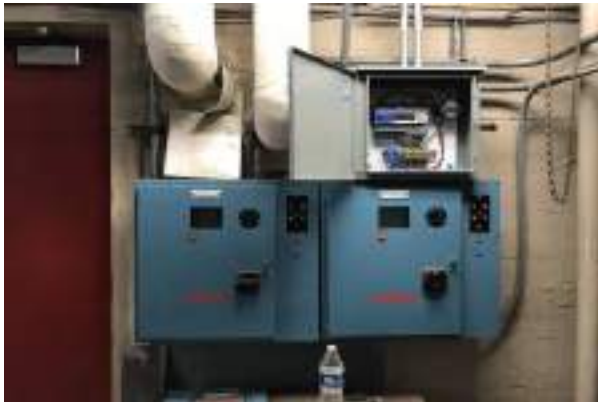
#69 BOILER CONTROLS
