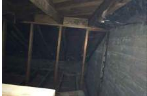
#44 BUILDING A INTERIOR ATTIC SPACE; INSULATION ON EXTERIOR WALL
