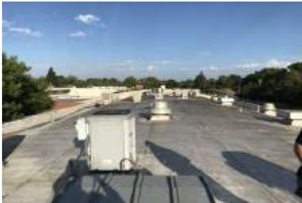
#21 ROTC (BUILDING C01) ROOF
