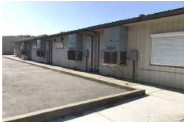
#16 BUILDING P02 REAR ELEVATION
