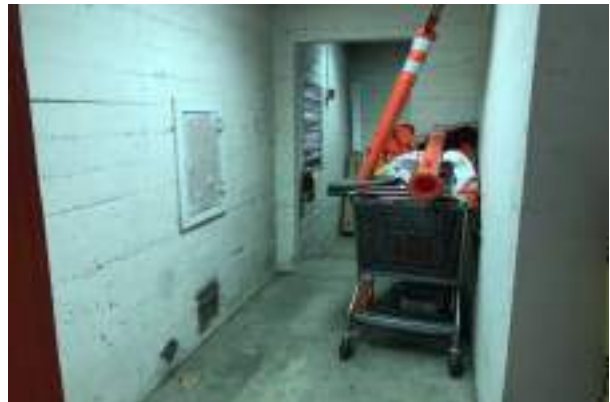
#36 BUILDING A BASEMENT
