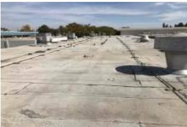
#15 BUILDING E ROOF, TYPICAL ROOFING FINISH
