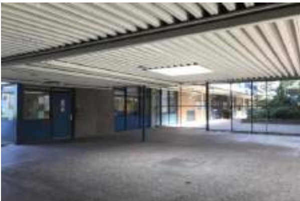
#5 BUILDING B AT OFFICES
