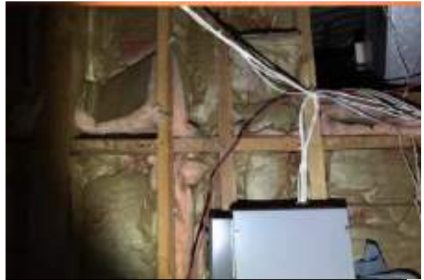
#20 BUILDING G INSULATION 3 1/2 INCH BATT
