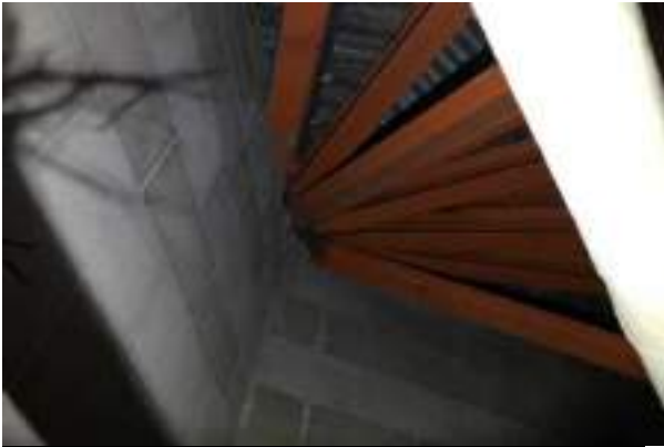
#19 BUILDING G STRUCTURE
