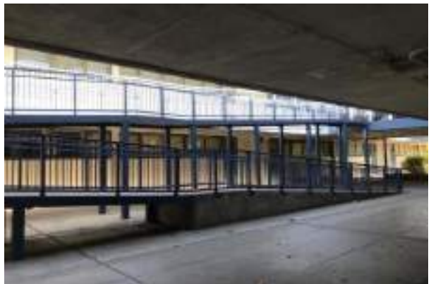
#6 BUILDING B RAMP
