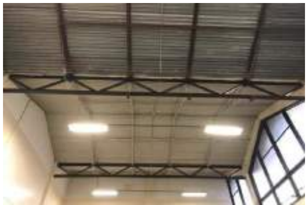
#16 BUILDING D STRUCTURE
