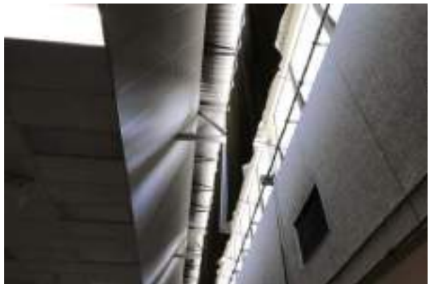
#18 BUILDING F STRUCTURE
