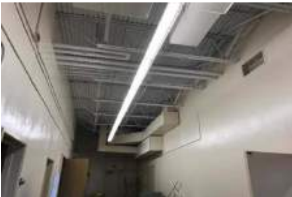
#17 BUILDING E STRUCTURE
