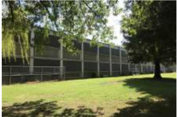
#2 FRONT ELEVATION-002 CLASSROOMS
