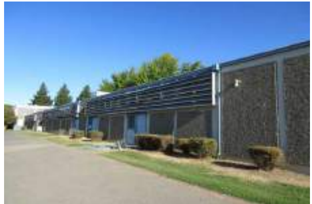
#10 FRONT ELEVATION-003 CLASSROOMS
