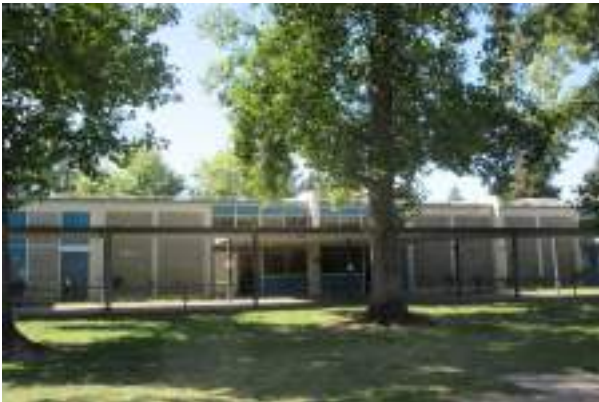
#9 FRONT ELEVATION-004 CLASSROOMS
