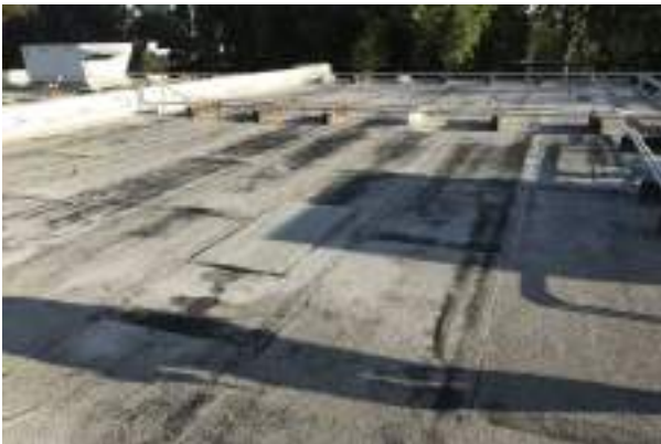
#23 TYPICAL MODIFIED BITUMEN ROOFING
