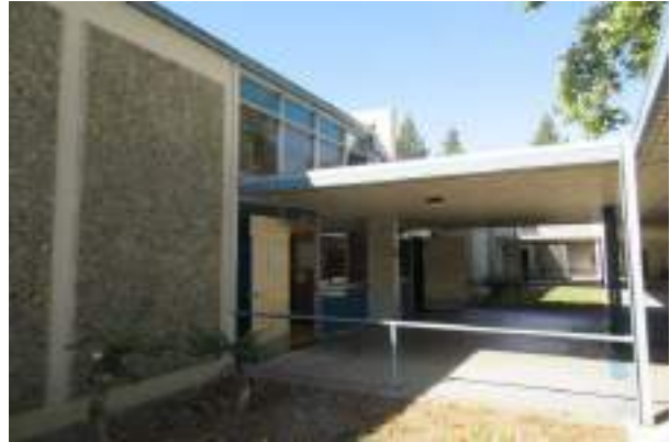
#26 TILT UP CONCRETE
