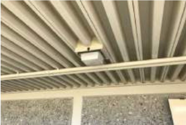
#25 SOFFIT COVERED WALKWAYS
