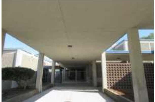
#20 SCHOOL COVERED ENTRY
