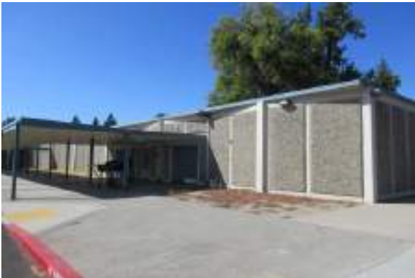
#3 FRONT ELEVATION-007 CLASSROOMS
