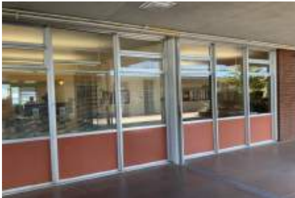
#9 CURTAIN WALL, ALUMINUM-FRAMED SYSTEM W/ GLAZING
