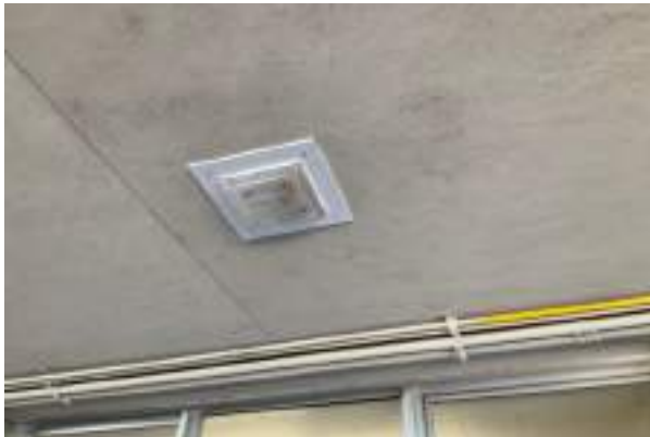
#39 COMPACT FLUORESCENT LIGHTING FIXTURE W/ ELECTRONIC BALLAST
