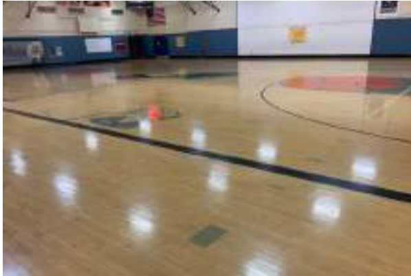
#19 INTERIOR FLOOR FINISH, MAPLE SPORTS FLOOR
