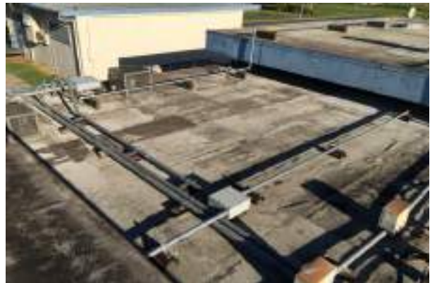
#12 MODIFIED BITUMINOUS ROOF MEMBRANE
