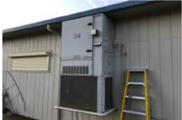
#32 GAS PACKAGE UNIT, WALL-MOUNT
