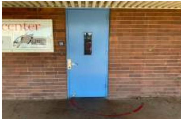
#6 EXTERIOR DOOR, STEEL
