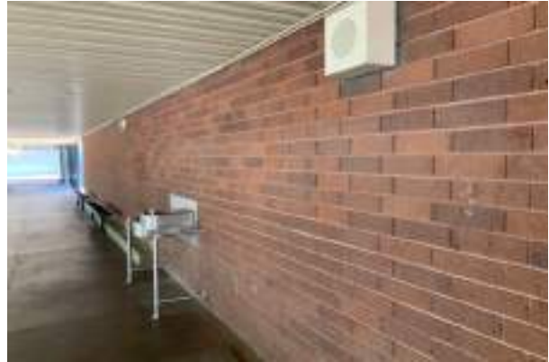
#8 EXTERIOR WALL, BRICK VENEER
