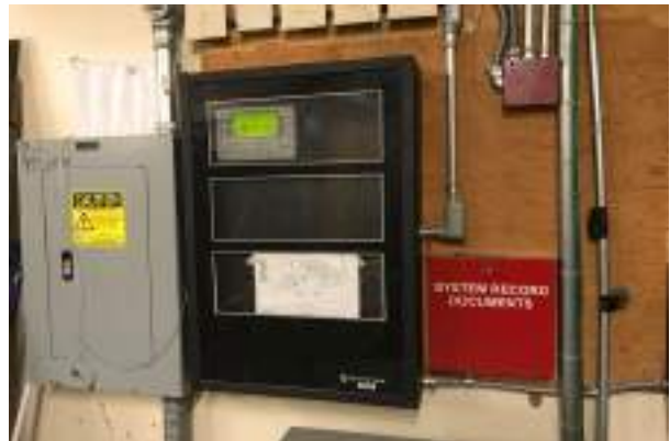
#42 FIRE ALARM CONTROL PANEL, BASIC/ZONED
