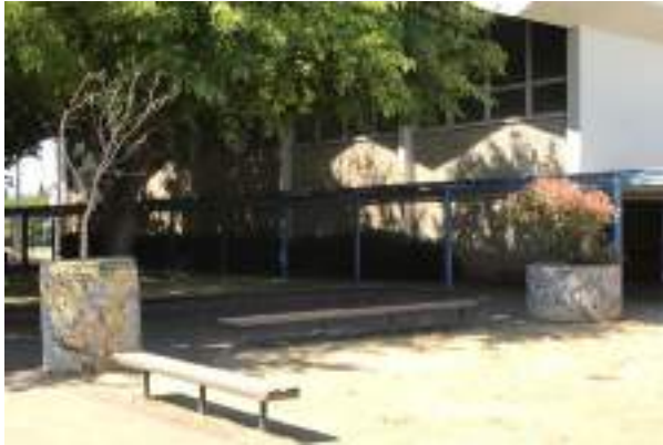
#7 GYMNASIUM EXTERIOR WALL
