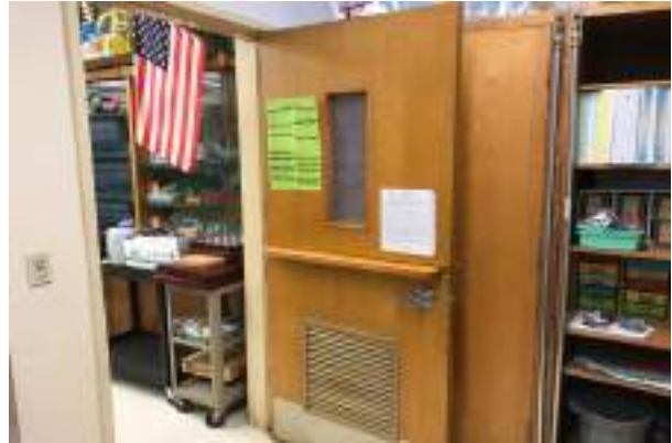
#14 INTERIOR DOOR, WOOD SOLID-CORE
