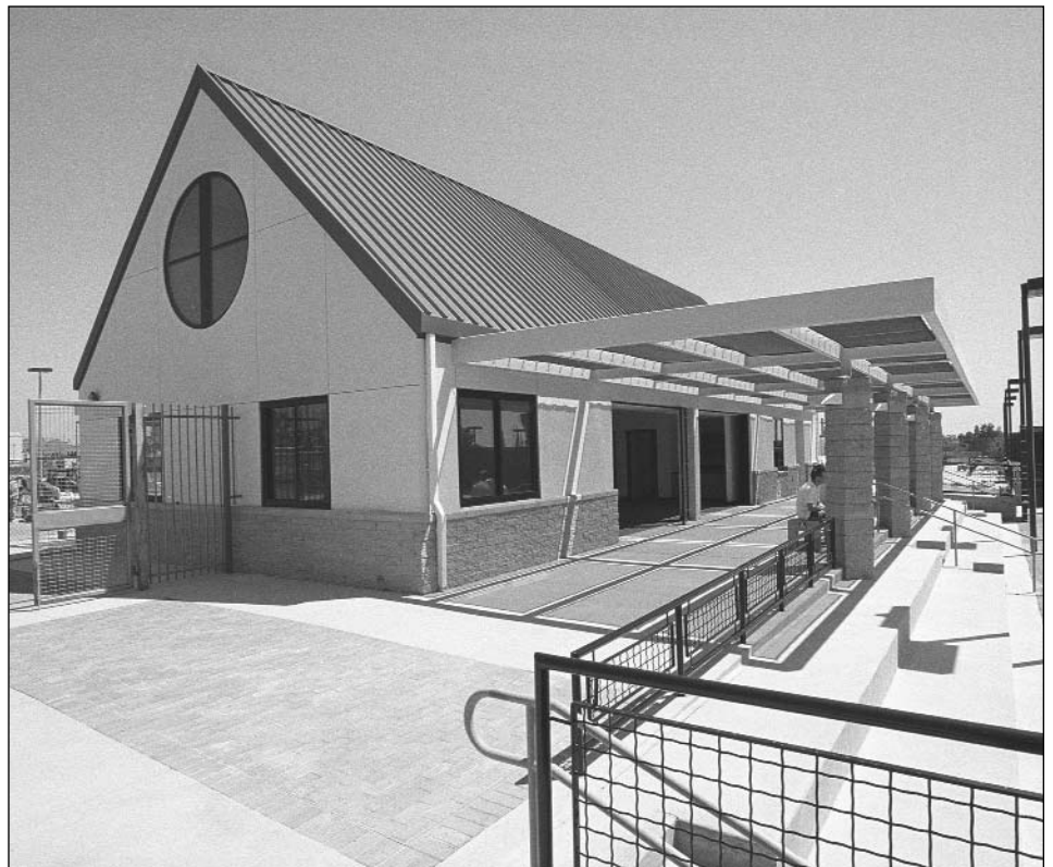
The Aztec Tennis Center operations building features office space, a lounge, team rooms and a kitchen.
