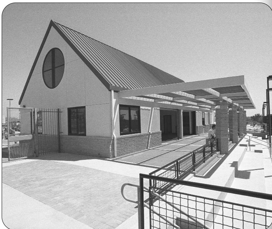
The operations building includes office space, a lounge, team rooms and a kitchen.
