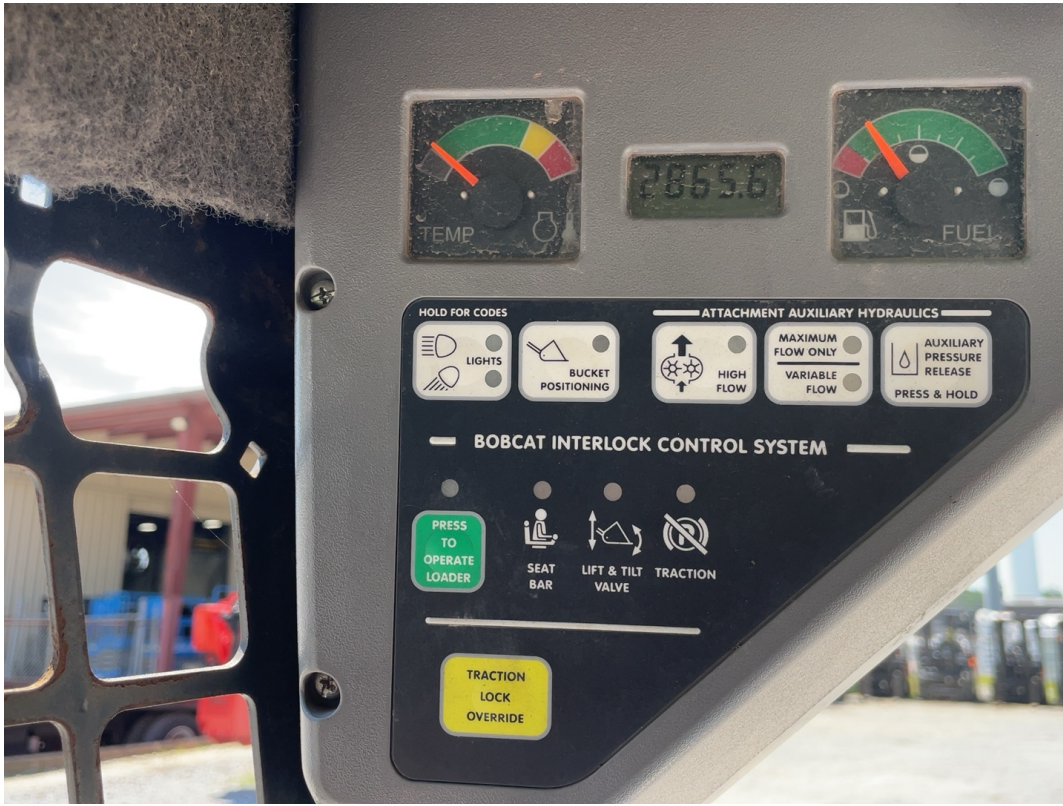
EMS Warning Lights / 05-15-2024
