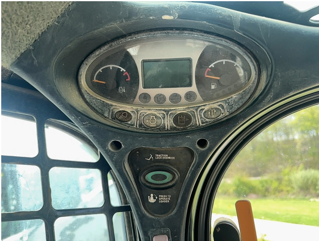
Switches and Controls / 04-26-2024
