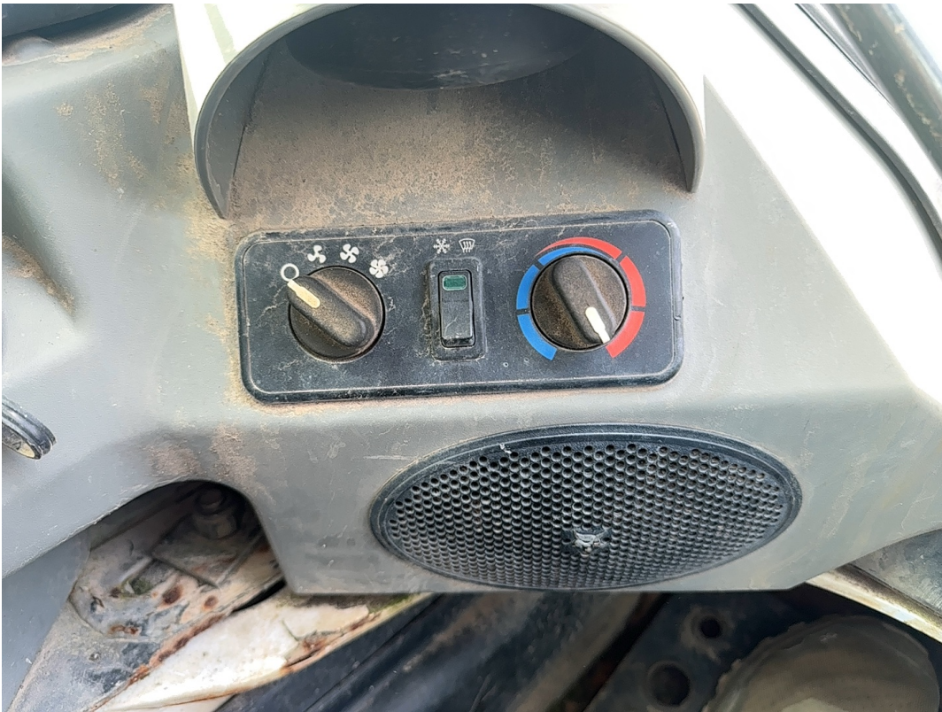
Switches and Controls / A/C / 04-26-2024
