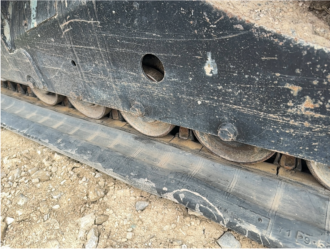
Left Track Condition / 04-26-2024
