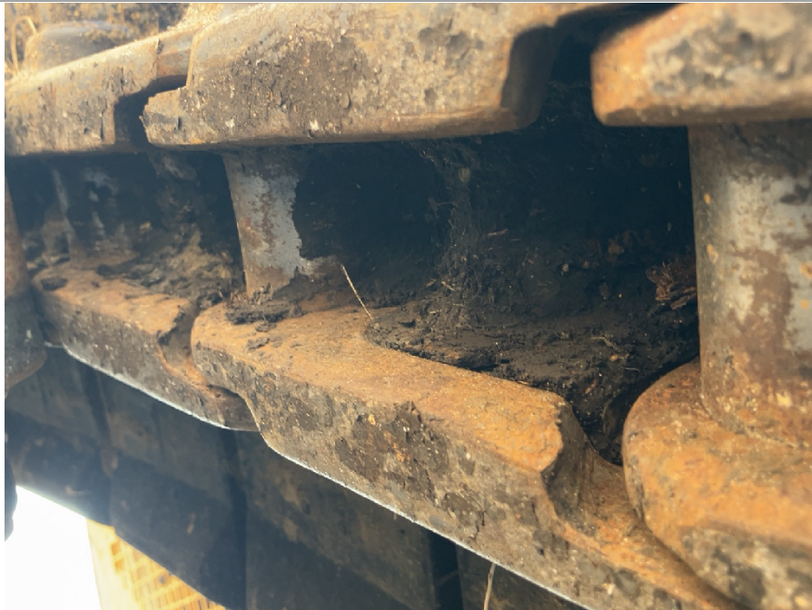
Right Track Condition
