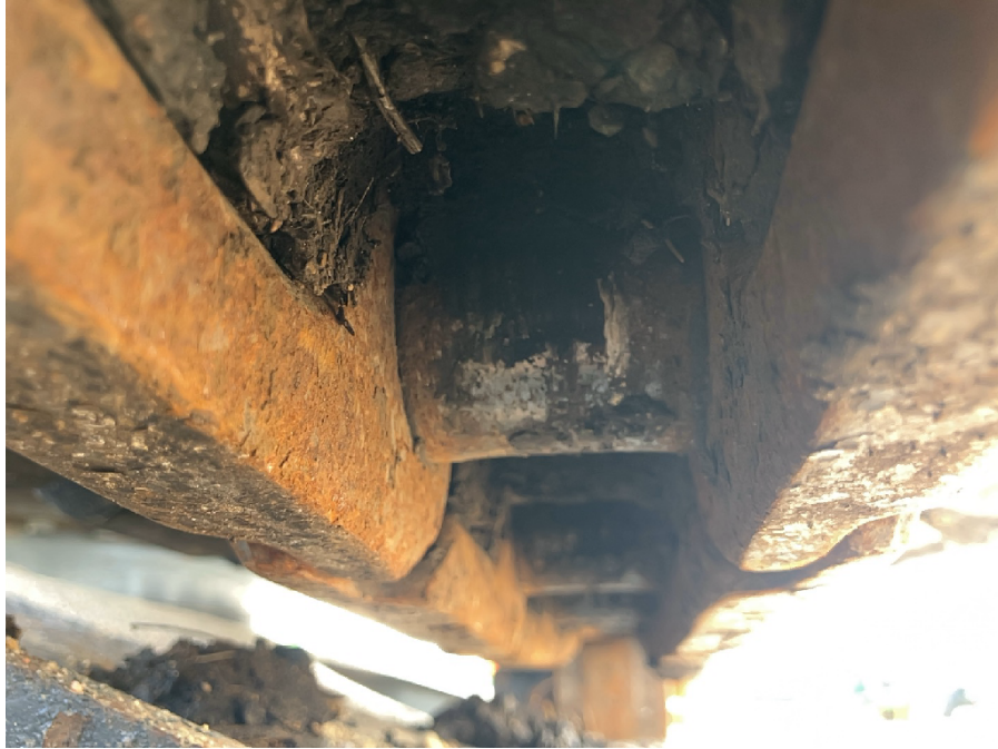
Left Track Condition
