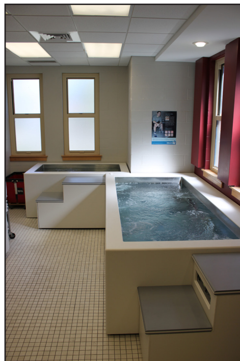
Brand new hot and cold tubs were installed in January 2013 inside the McIntosh Building training room, which should assist in the prevention and treatment of injuries.
