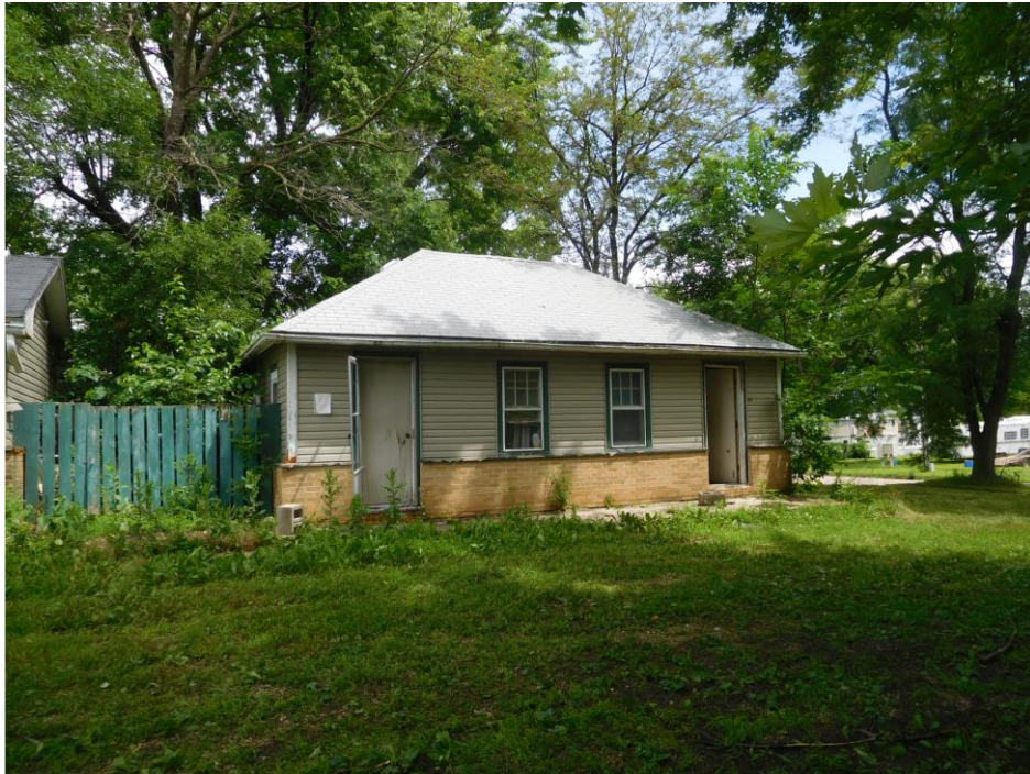
PHOTO 7: Overview of Northeastern units. The former two units were converted into one.
