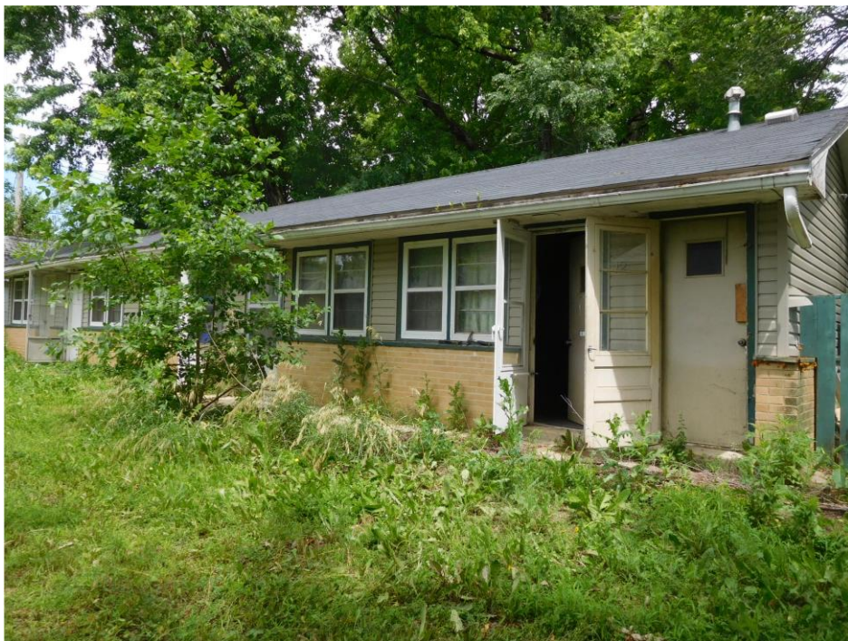
PHOTO 8: North Central units. Many units were modified with kitchenettes added and many units combined.
