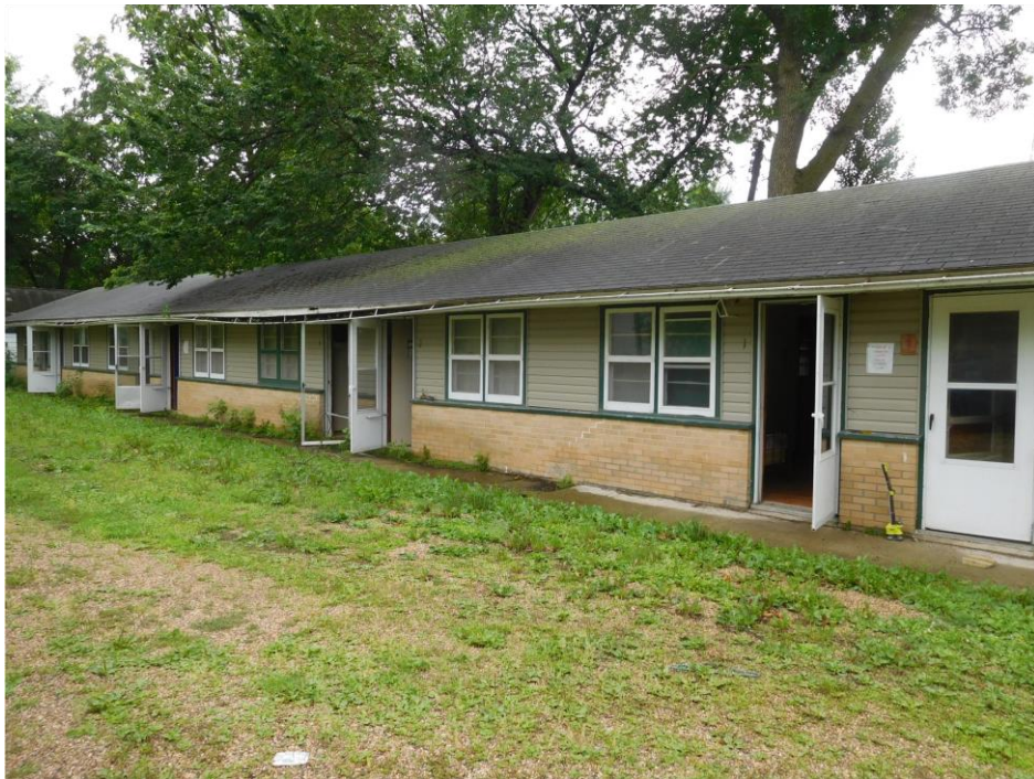
PHOTO 1: Exterior overview of the Northern face of the Southern Units.
