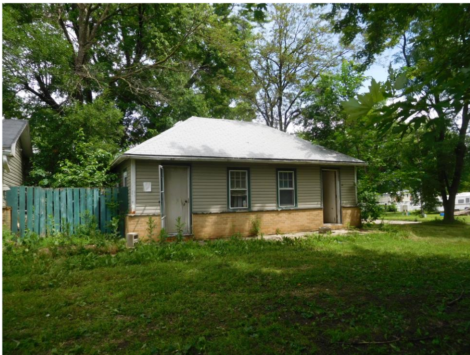
PHOTO 2: Exterior overview of the East duplex's Southern elevation. Two units are now one.
