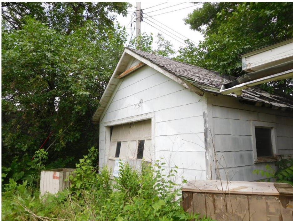
PHOTO 4: Western garage with asbestos containing transite siding on the exterior.
