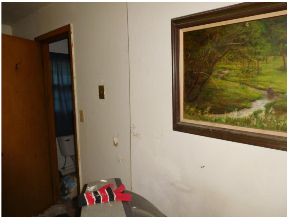
PHOTO 10: Interior Unit #12, asbestos containing wall materials.
