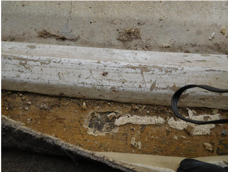
PHOTO 9: Unit 9, under carpet, Asbestos Containing Floor Tile and Mastic adhesive.
