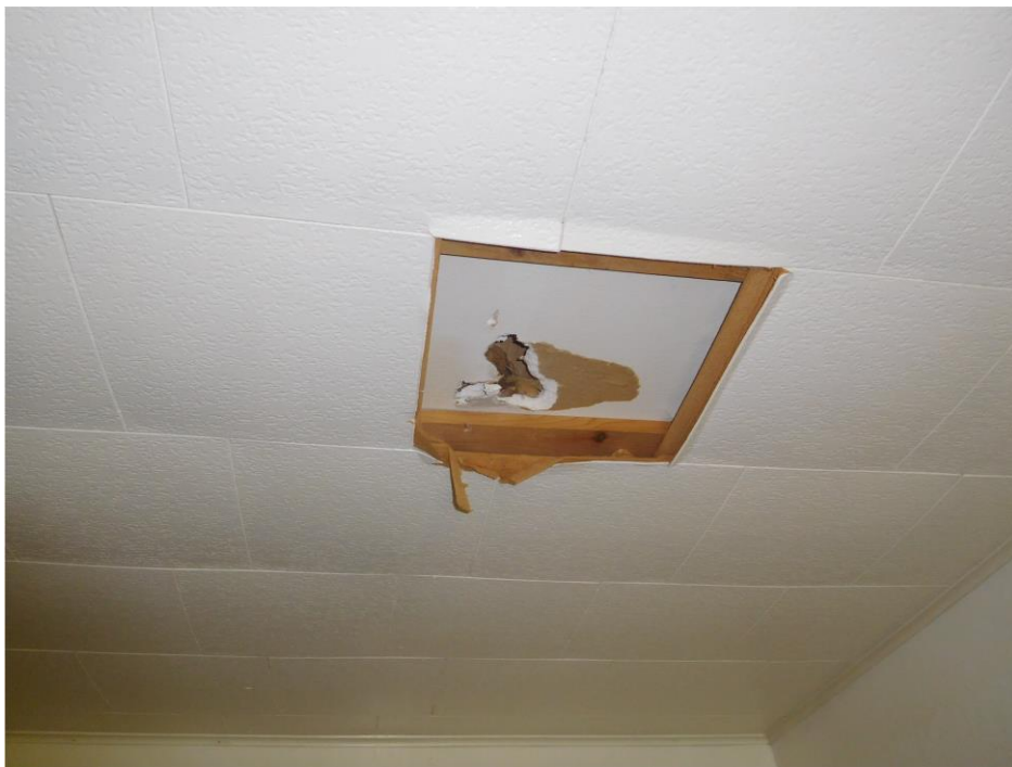
PHOTO 6: Interior of Unit #1, ceiling system. Non-asbestos ceiling tile with asbestos containing drywall materials ( asbestos found in the joint compound).
