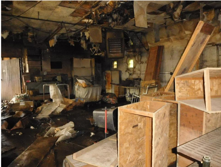
PHOTO 3: Interior center section of main building. Overview of separation boxes, fallen ceiling tile and exposed insulation.
