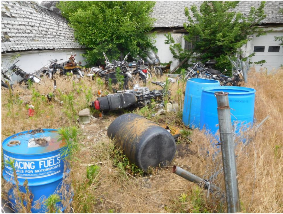
PHOTO 9: South exterior side of West building. Laydown area for motorcycles and parts. Note: drum marked racing fuels. Note: top layer of roofing on Main building is asbestos containing .
