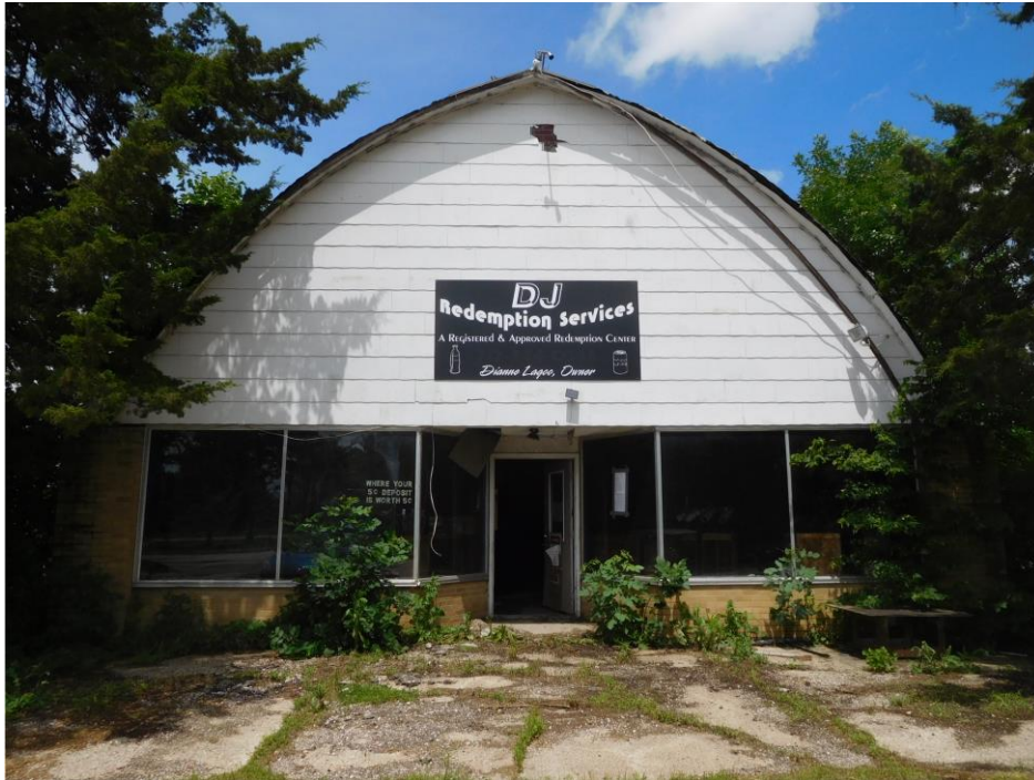
PHOTO 1: Address side of the former DJ Redemption Services Building. Note: asbestos containing siding on building.
