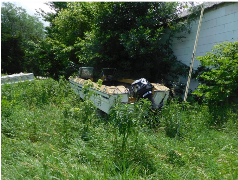
PHOTO 10: East yard area of main building. Overgrown vegetation covers boat, household furniture, windows, awnings, etc. Note: asbestos containing siding on East exposure north end of main building.
