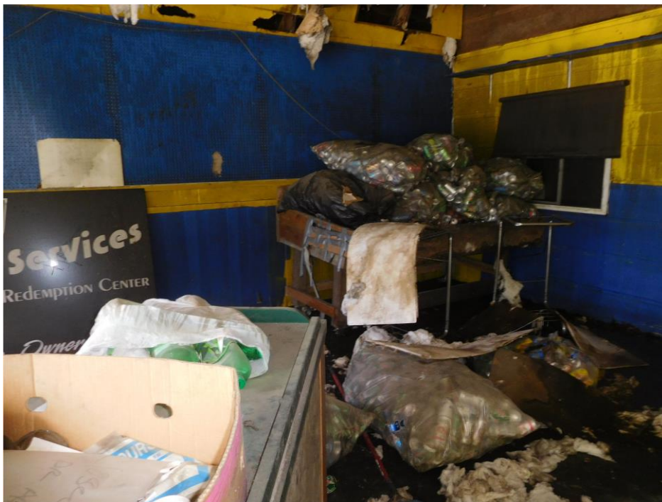
PHOTO 2: Interior of office area of property. Building has aluminum cans and assorted metals.
