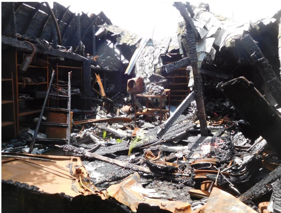
PHOTO 6: West building, East end. Extensive fire damage. Motorcycle engines and parts. No salvage.
