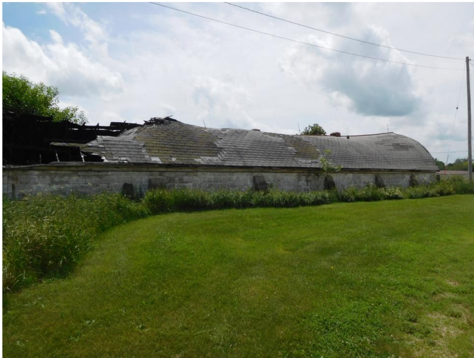
PHOTO 7: Overview of West building with East end having the fire. Non-asbestos roofing on West building.
