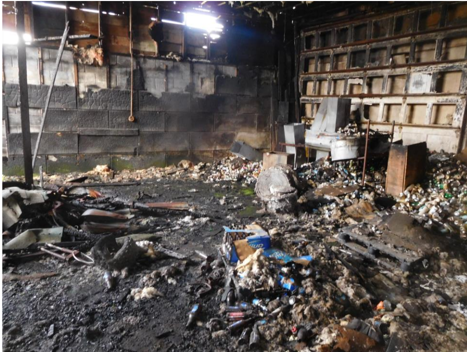
PHOTO 5: North section of main building. Extensive fire damage to structure. Assorted debris and aluminum cans.
