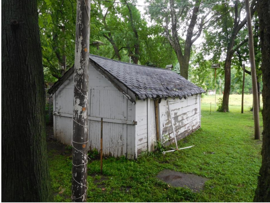
PHOTO 3: Exterior overview of the South and West elevations of the garage.
