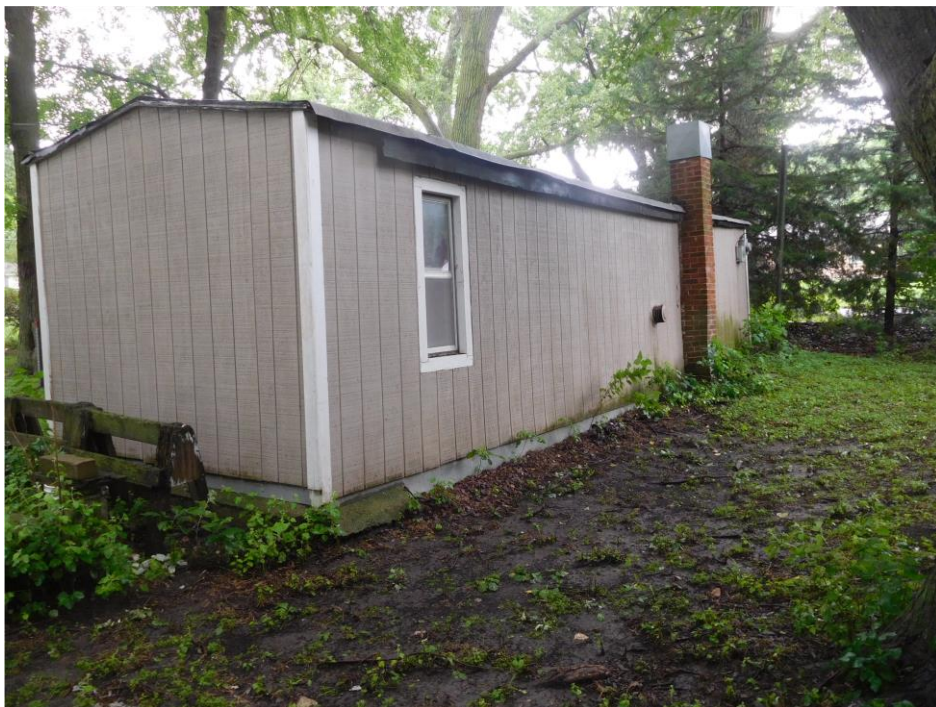
PHOTO 2: Exterior overview of the North and East elevations of the house.
