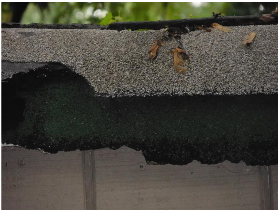
PHOTO 8: Roof of house. Multiple layers of rolled shingles and tars. Original rolled roofing with tar and the second layer of the four layers are asbestos containing .
