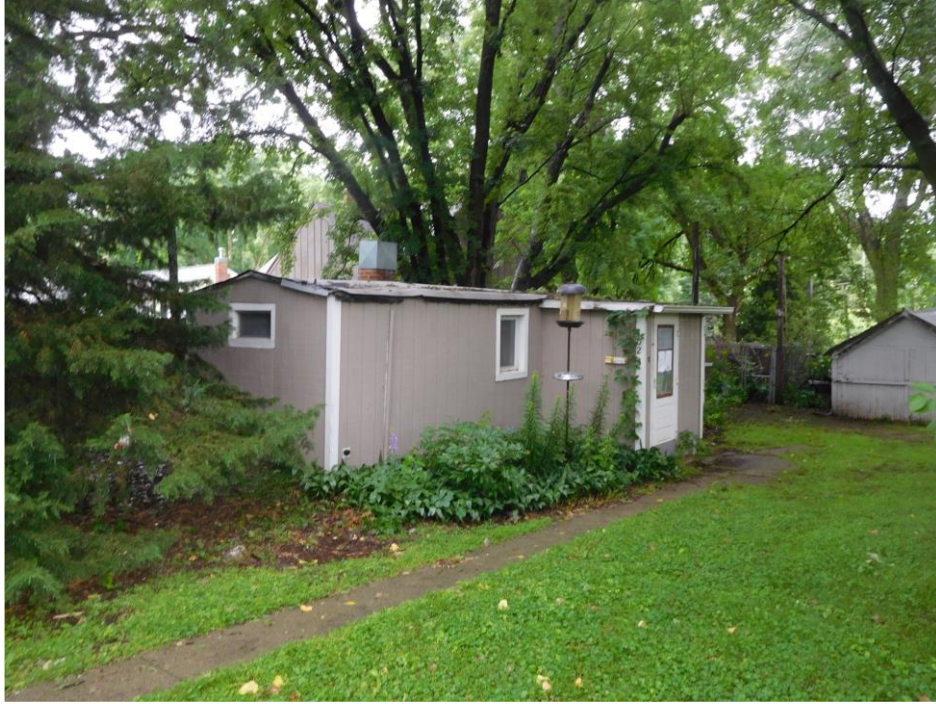
PHOTO 1: Exterior overview of the South and West elevations of the house.
