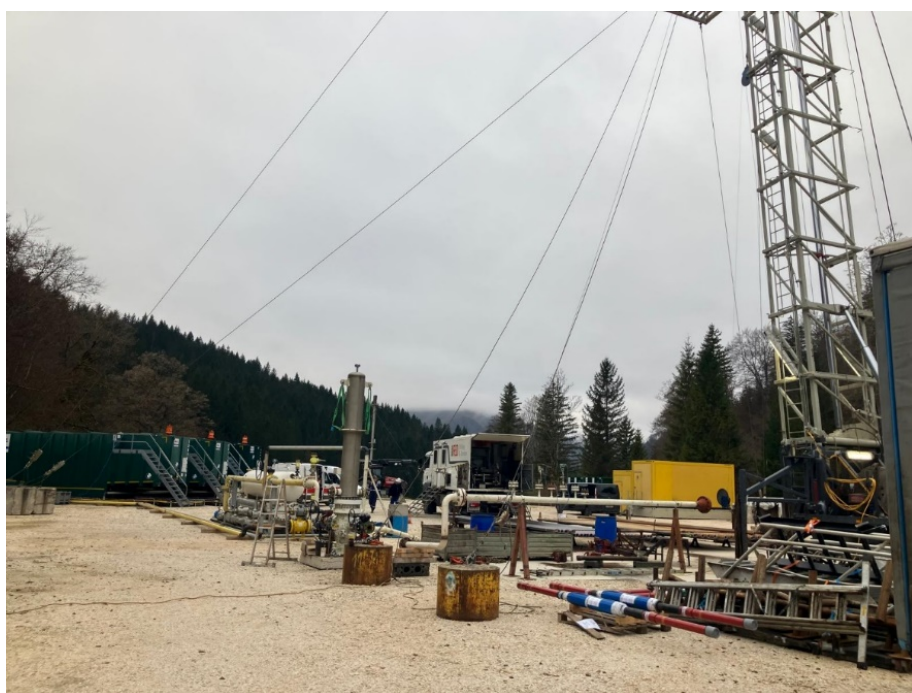
Well completion operations and Flow Testing Facilities set up at the Welchau-1 well location
