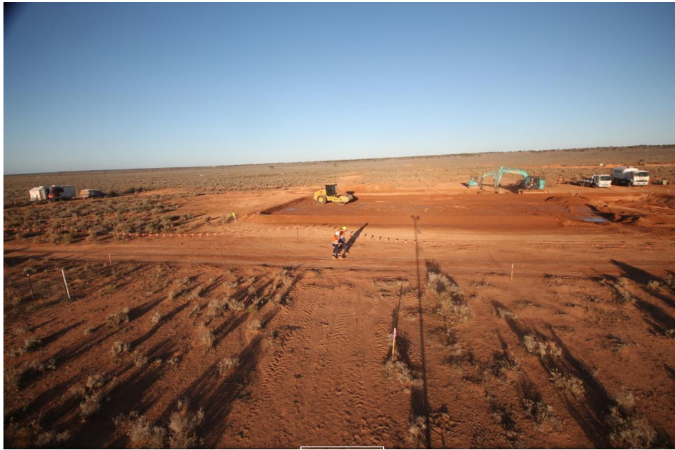
Figure 1. Construction commencing on the Field Recovery Trial
