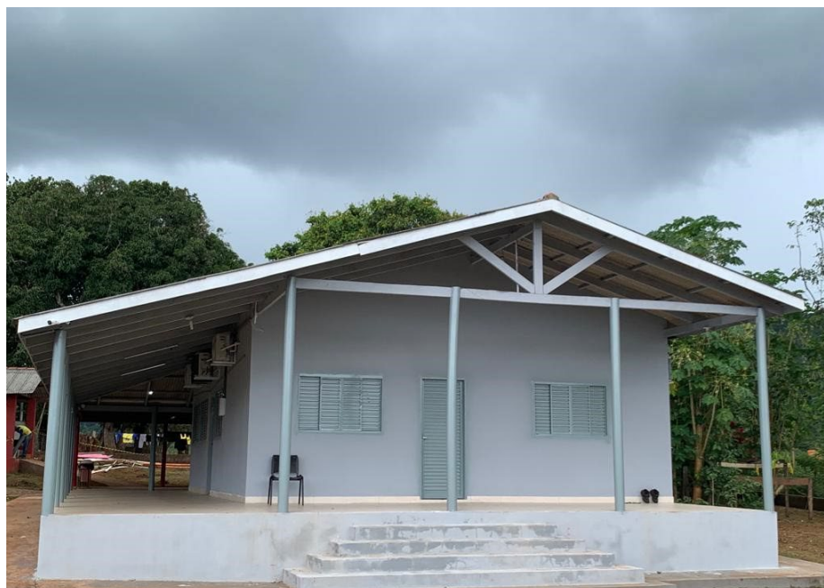
Figure 6: New On-site Accommodation at Jaguar
