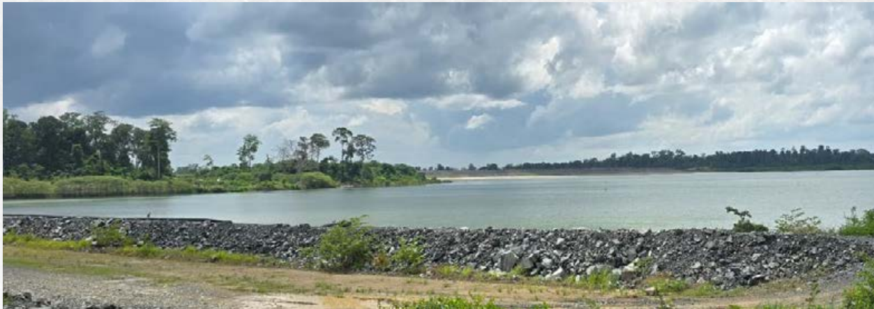
Figure 38 | Tailings Storage Facility at Okvau
