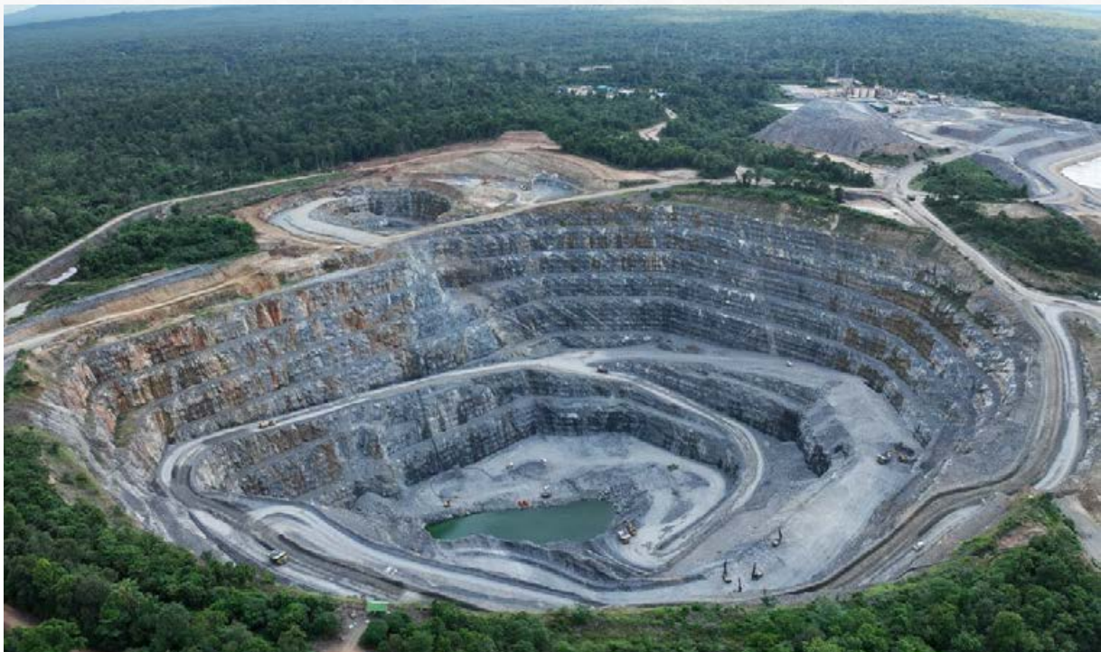
Figure 4 | Okvau Open Pit at July 2025
