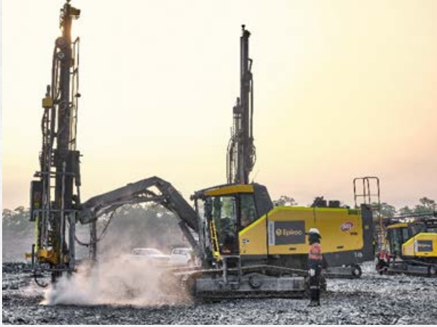
Figure 5 | Epiroc T-45 Blast Hole Drills at Okvau
