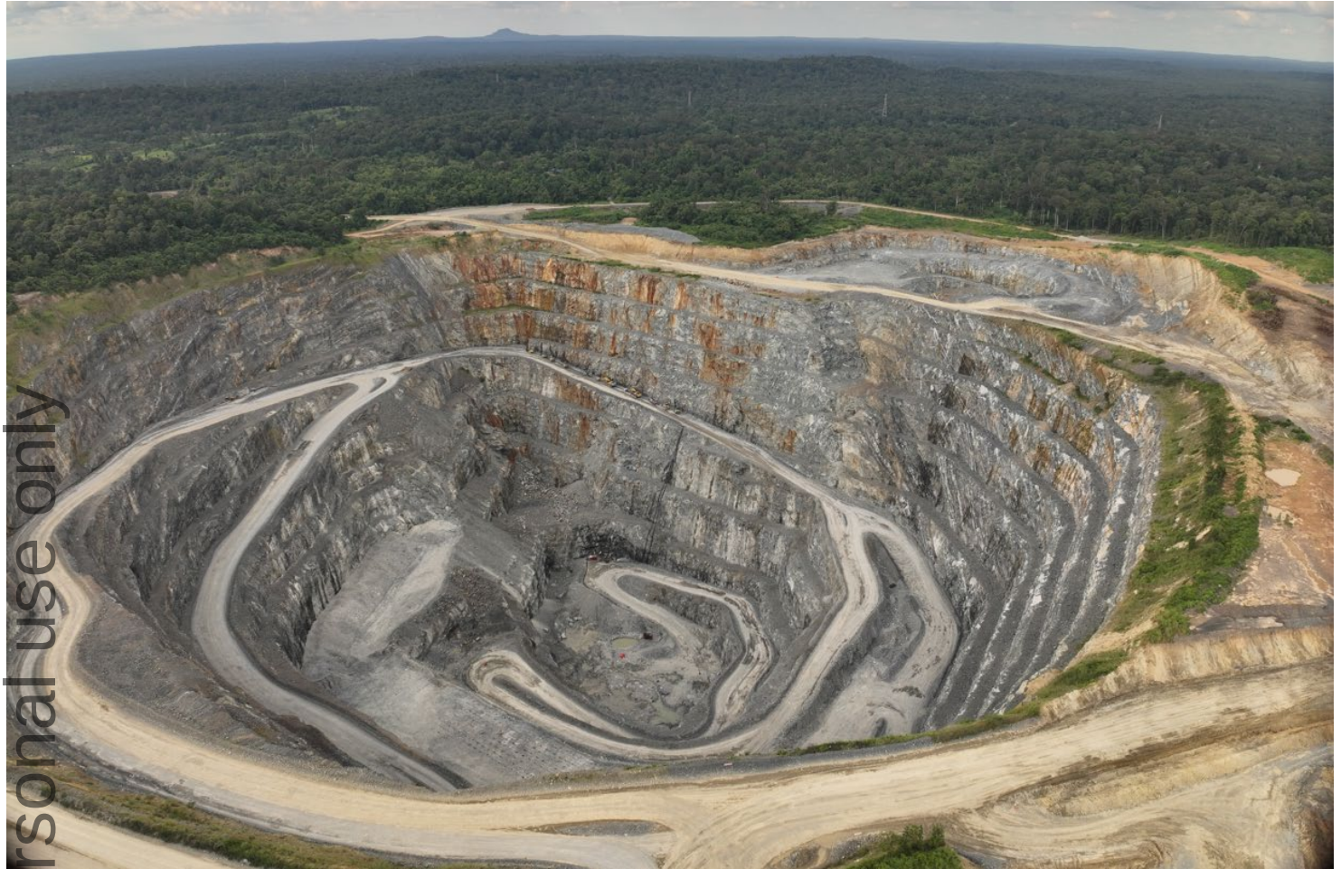
Figure 1 | Okvau Open Pit – October 2025
