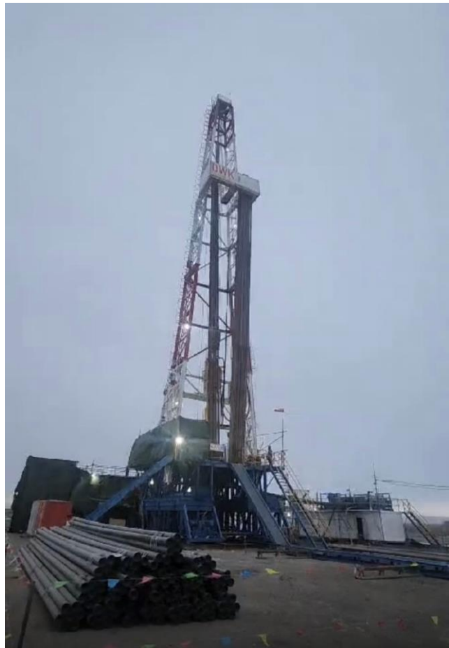
Figure 2: DWK Drill Rig on location at Production Well Two, Red Lake Gas Field, South Gobi
