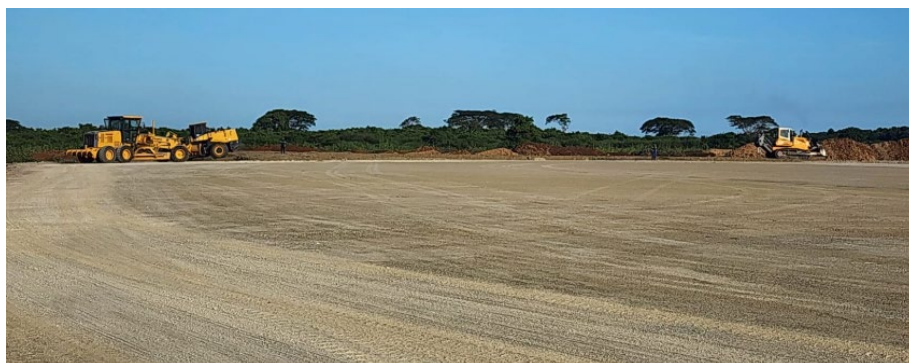
Figure 3 - Construction of pad for Amistad-3 was completed.
