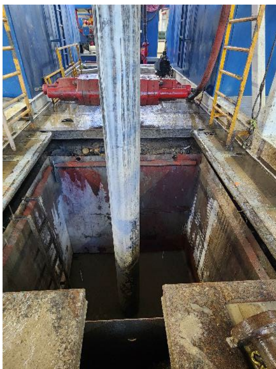
Figure 1 - Surface casing set in place
