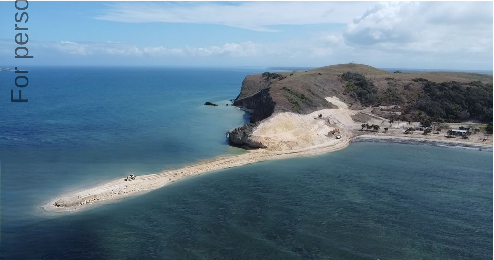
Stage 1 of the wharf under construction
