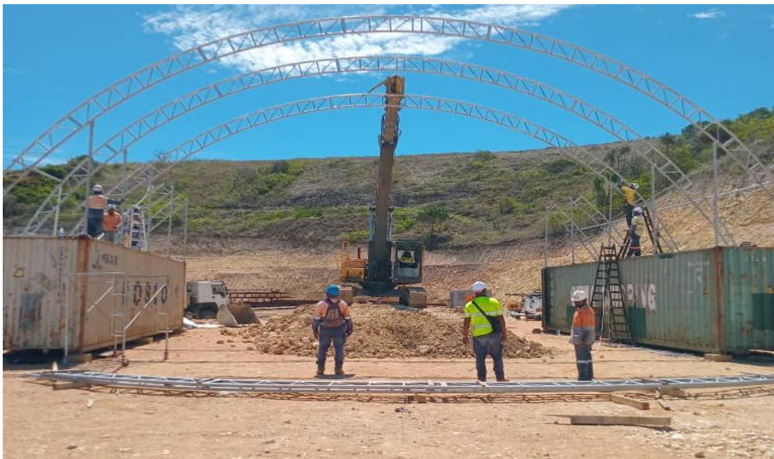
Construction of Workshop Area
