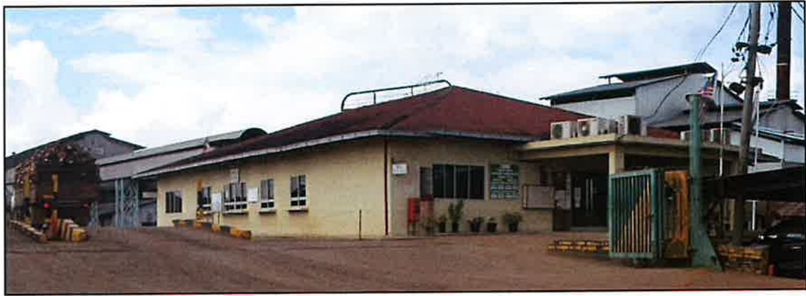
VIEW OF THE OFFICE BUILDING
