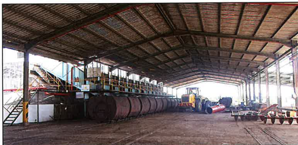
VIEW OF TRANSFER CARRIAGE AND LOADING RAMP
