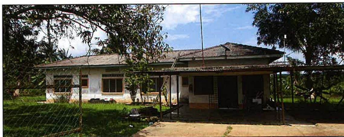
VIEW OF MILL ASSISTANT MANAGER'S BUNGALOW
