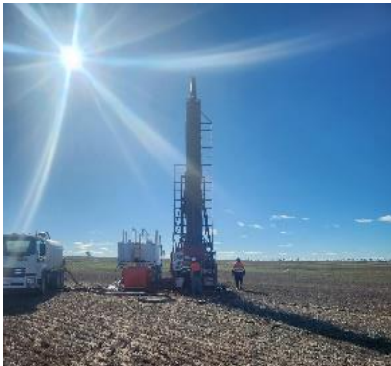
Photo 3: Drill Rig Alford West Project
