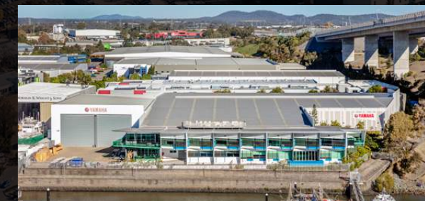
69 RIVERGATE PLACE, MURARRIE QLD 2
