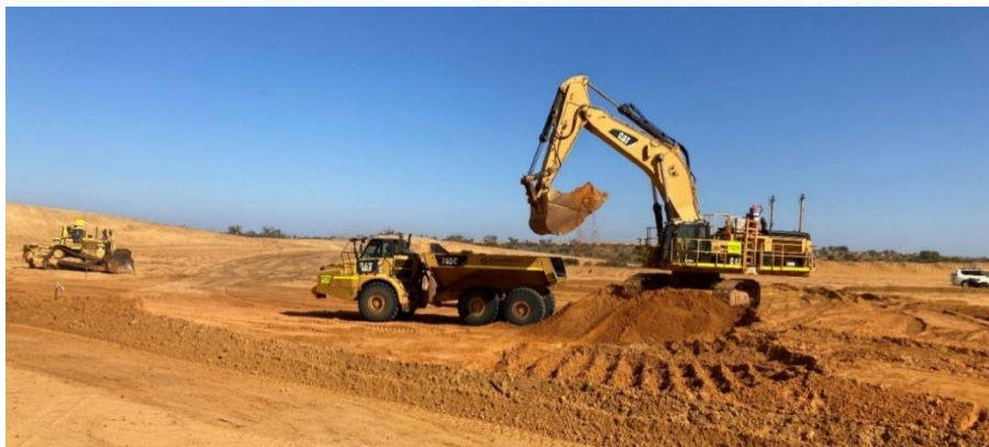
Figure 3 – Breaking ground at Ambassador North pit (11 December 2021)
