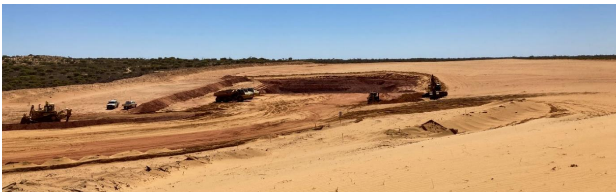
Figure 1 – Ambassador North pit ramp excavation
