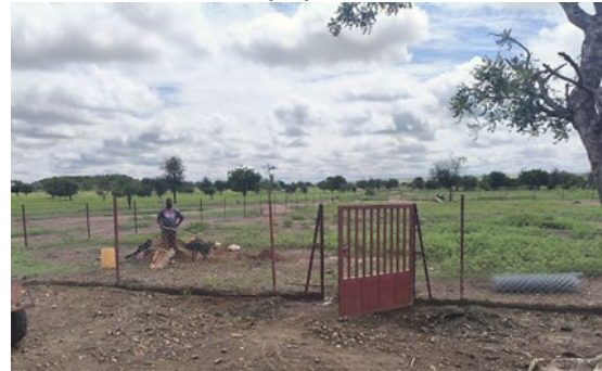
Fence construction at market garden extension project
