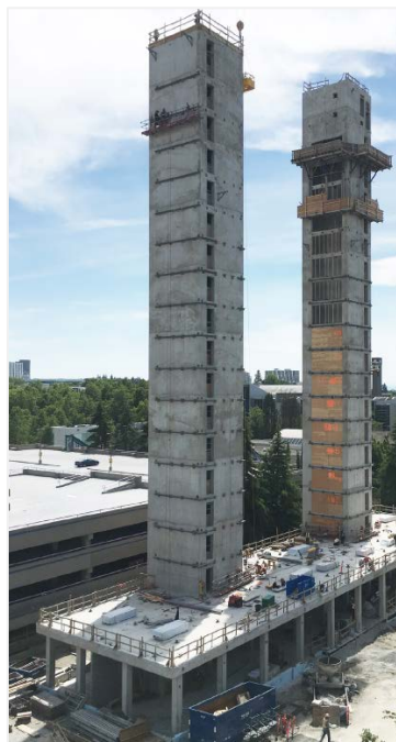
Figure 12: On-site Concrete Components
