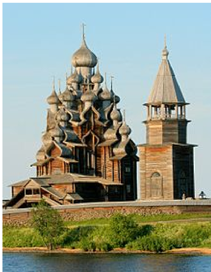
Church in Kizhi, Russia (constructed entirely out of wood--log building technique)
