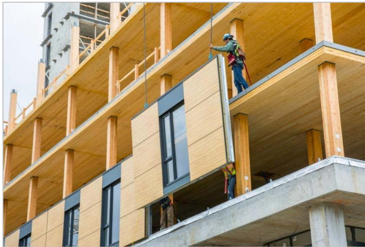
Figure 15: On-site Prefabricated Envelope Erection
