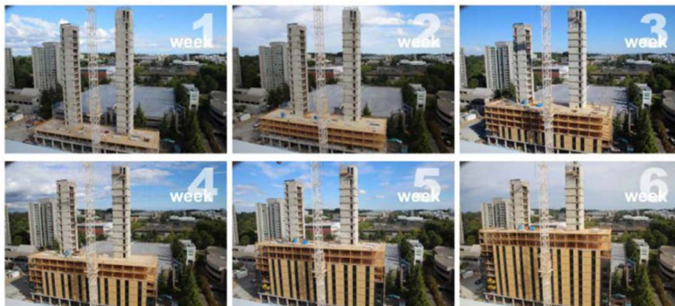
Figure 14: Progress across Six Weeks for Mass Wood and Envelope
