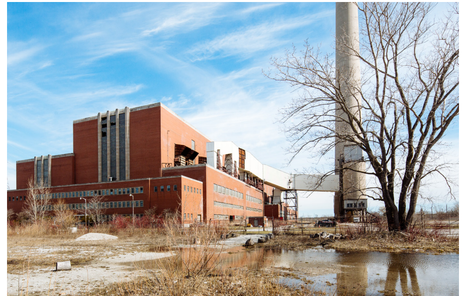
The Hearn Power Station, opened in 1951, was the site of Canada's first 100 MW steam turbo-generator set.
