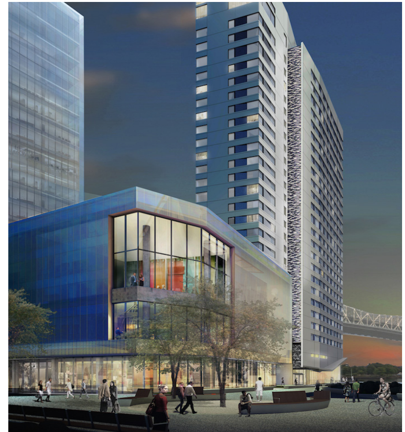
At 26 stories, Cornell Tech's residential tower is the tallest Passive House building ever built. It is projected to achieve a 73% reduction in overall energy consumption compared to the median of comparable New York City buildings. Although Passive House added 5-10% to the cost of this building, key cost drivers were identified as sources of future innovation and savings, such as developing new techniques for testing how well the building is sealed. Credit: Cornell Tech
