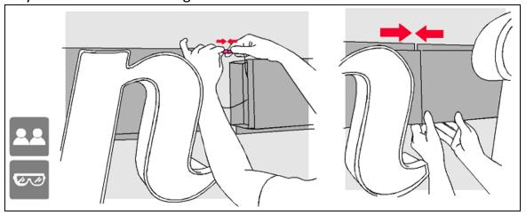
Mount each additional raceway to the wall after leveling to the raceway directly before it. Continue installing all the mounting screws through the top and bottom flange.
