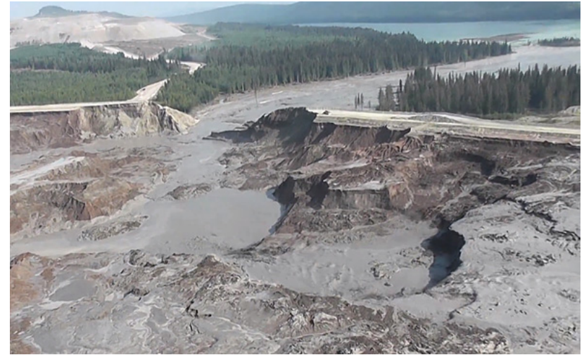
Mt. Polly tailings dam collapse
