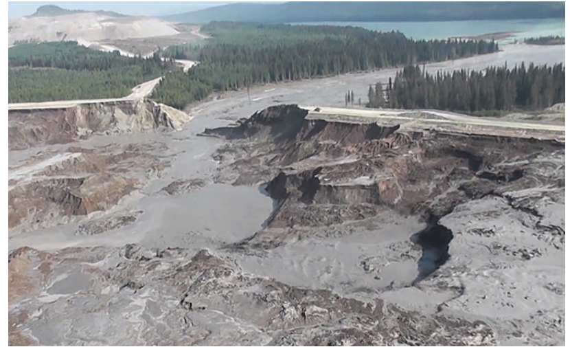
Mt. Polly tailings dam collapse
