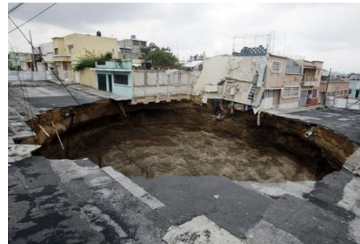
Subsurface voids
