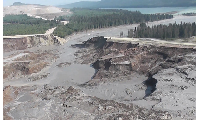
Mt. Polly tailings dam collapse
