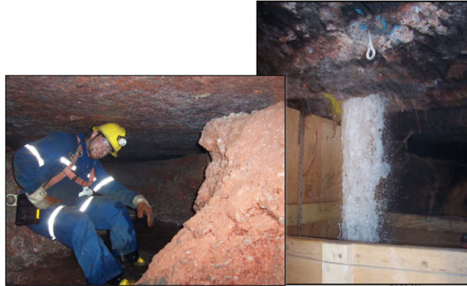
Fig. Inflow problems in a mine
