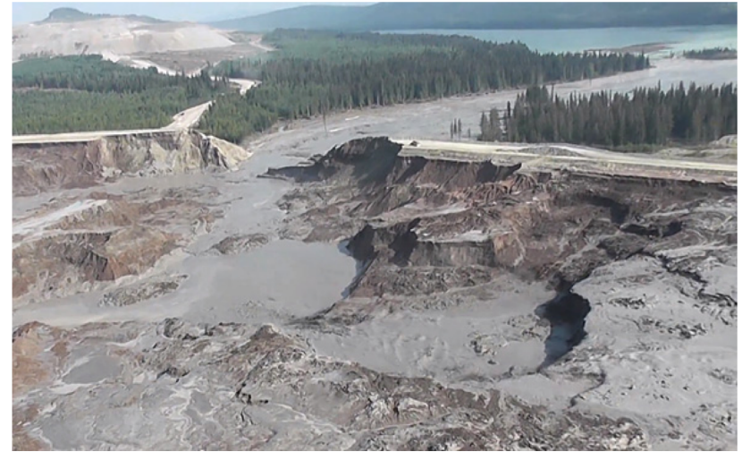
Mt. Polly tailings dam collapse
