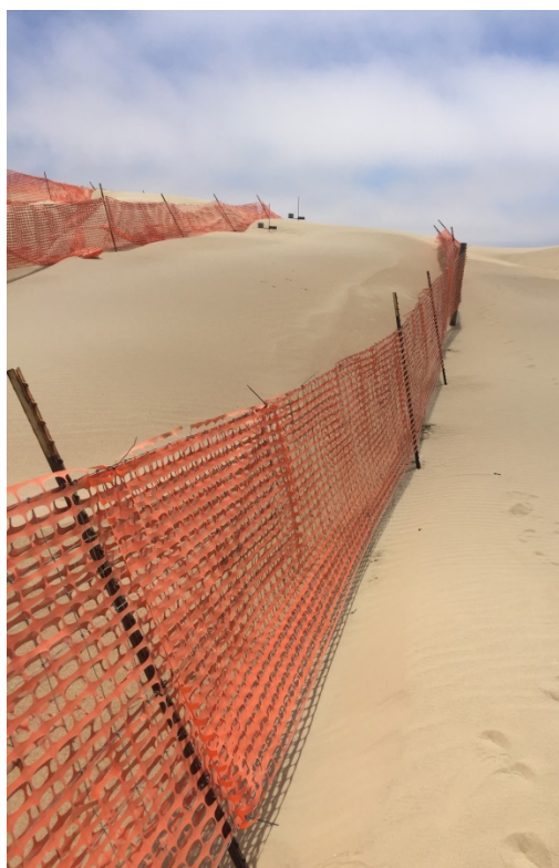
Exhibit 3. 2018 wind fencing projects installed at Oceano Dunes SVRA. Partially buried fencing requiring maintenance is visible in the top and lower right photographs.
