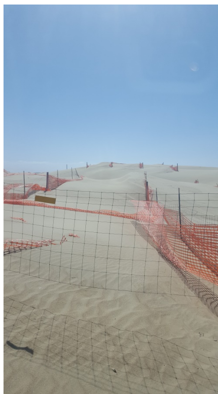
Exhibit 3. 2018 wind fencing projects installed at Oceano Dunes SVRA. Partially buried fencing requiring maintenance is visible in the top and lower right photographs.
