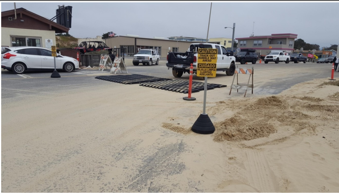
Exhibit 4. Pier Avenue Trackout Mats.
